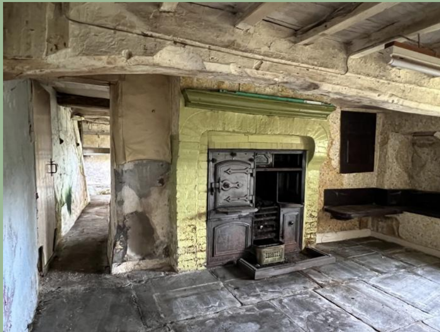
Caption: the firehouse of the 17 th Century Scrithwaite Farmhouse, Lickle Valley, with its large bressummer beam, inserted range, spice cupboard and blocked fire window.
