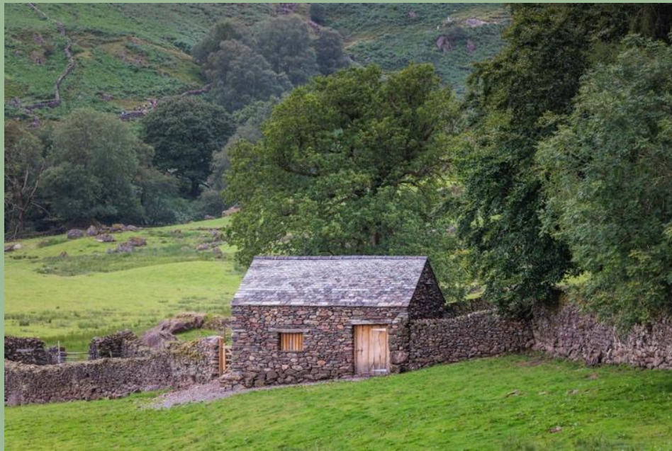
Caption: Far Easedale Barn post-repair, 2024
