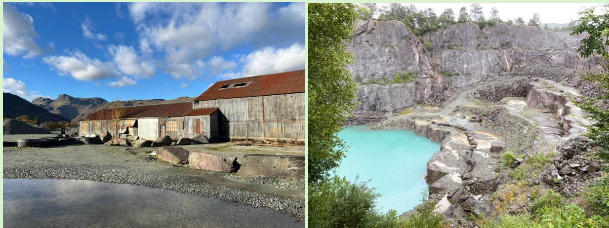
Photos: Elterwater Riving (processing) Sheds and the Quarry. © R Lord.
