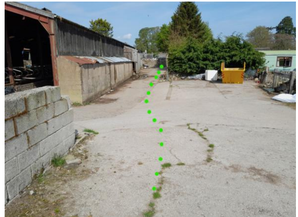
Looking towards the road and Point D
