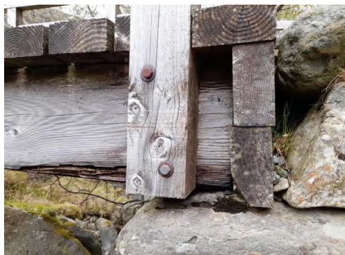
Rot of the upstream beam
