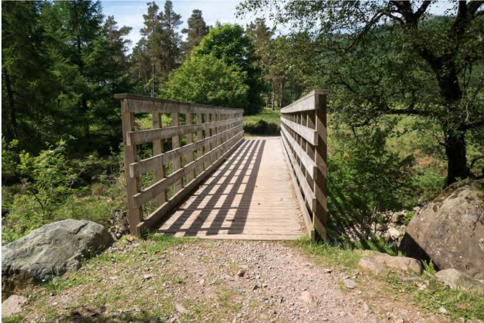
Galloway Bridge in 2018
