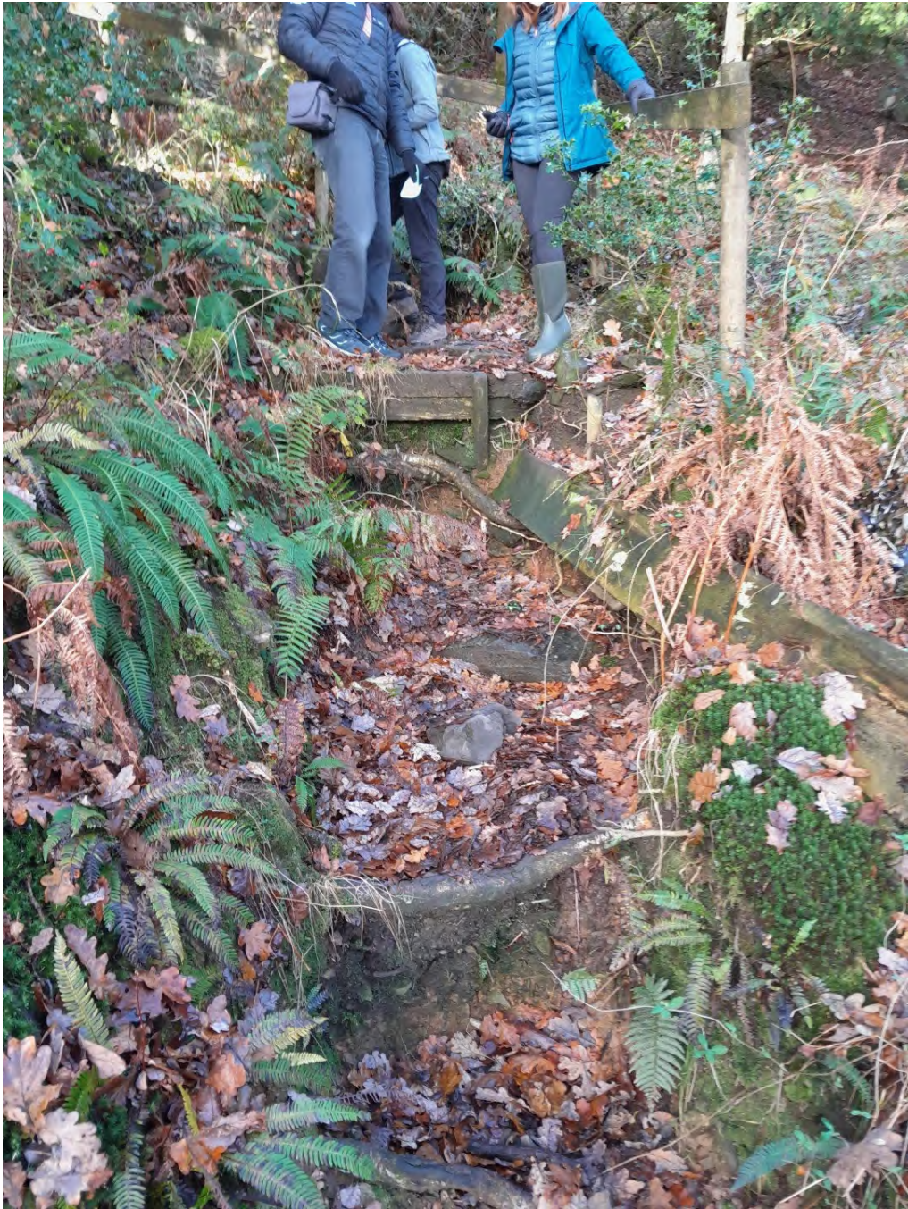
An example of some of the old steps that have now been replaced (the top step is higher than it looks)
