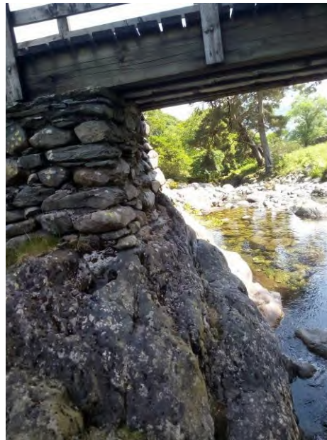
Abutment and beams
