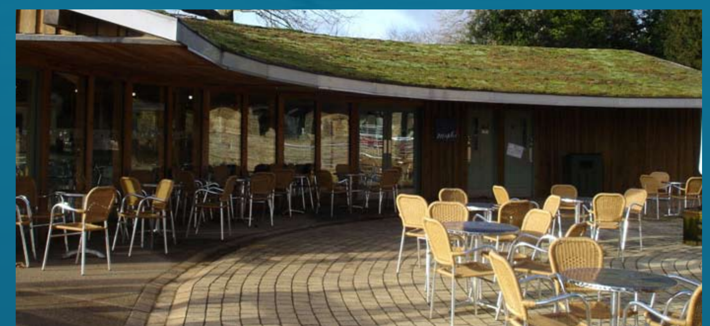
New development, known as 'The Courtyards' could be delivered on the existing tennis court, Tourist Information and Toilet site
