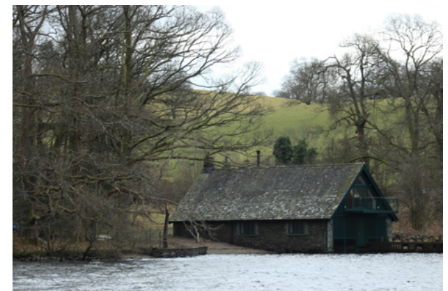
6.6.4 Larger boathouse with decking
