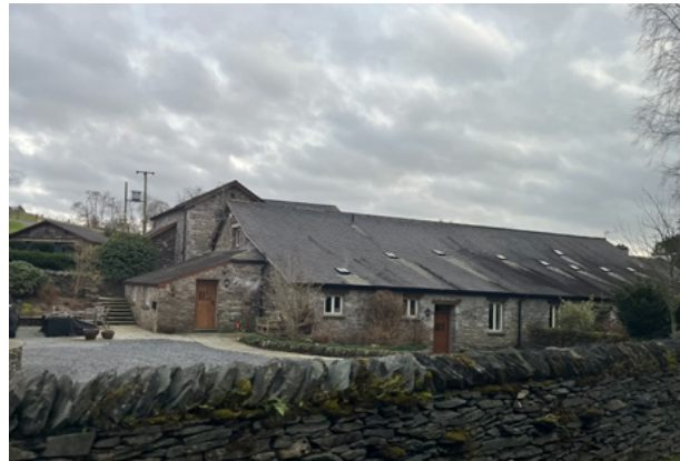
5.1.3 Vernacular agricultural building converted to residential use
