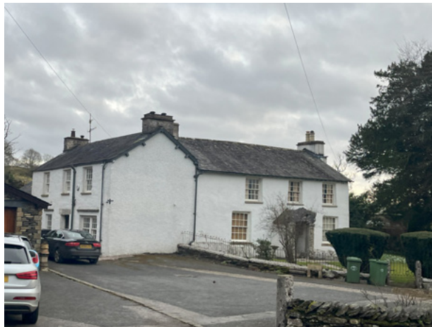
6.1.3 Classicised double pile farmhouse
