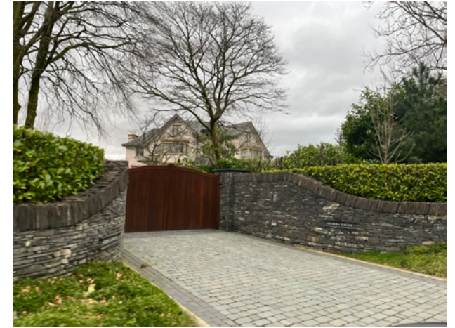
7.2.13 High boundary wall and gates to properties
