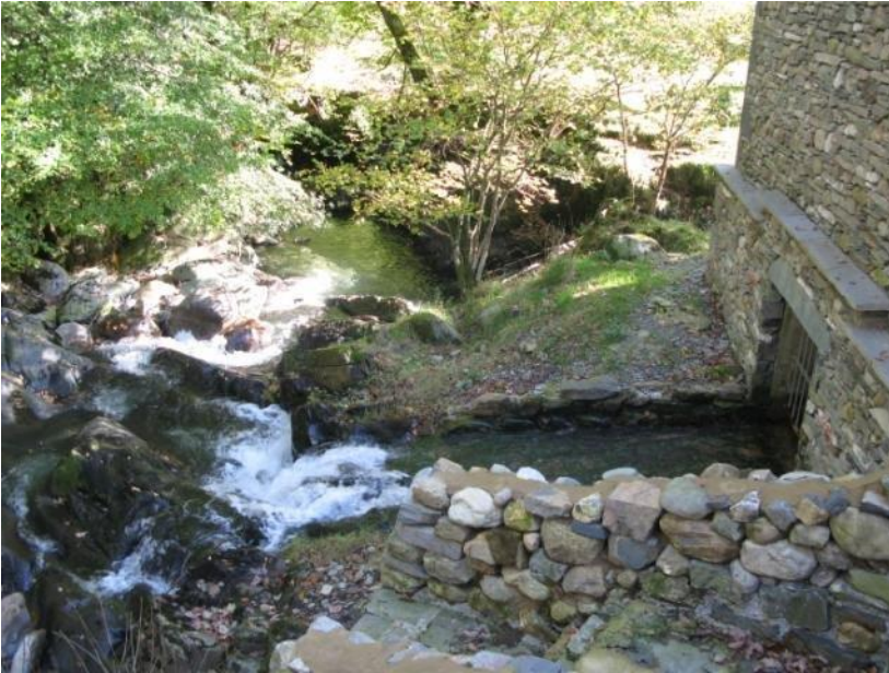
Church Beck hydro scheme, Coniston
