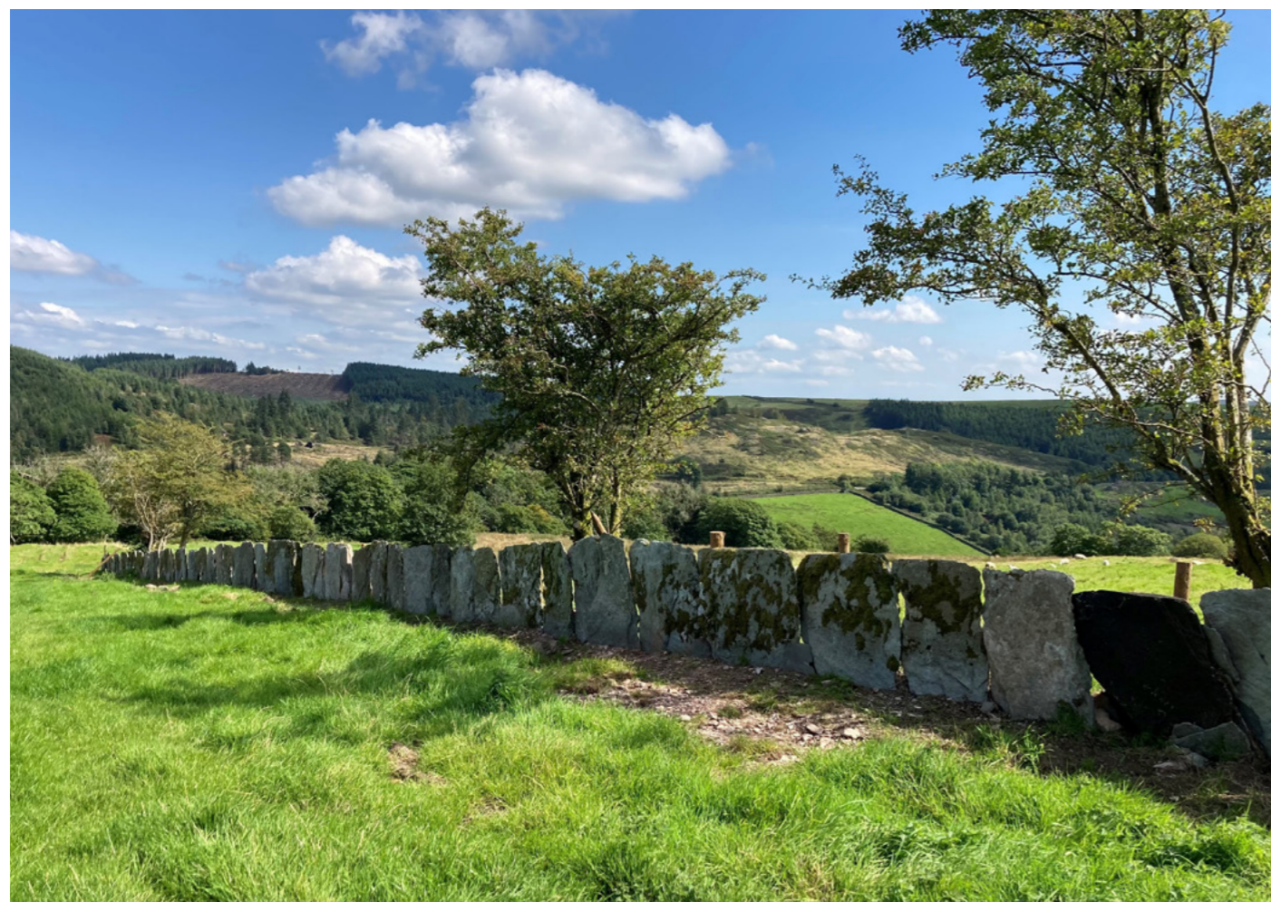
Shard fencing in the Lickle Valley which is being restored with FiPL funding
