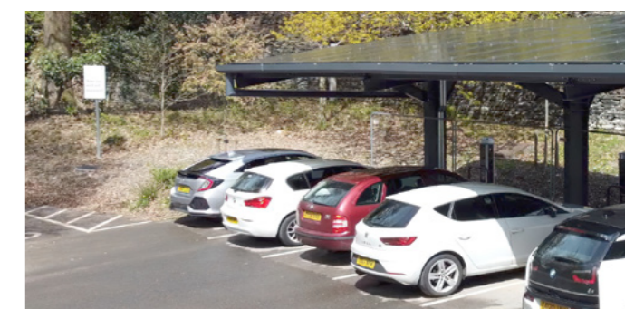
Electric vehicle charging station powered by solar panels at Brockhole on Windermere
