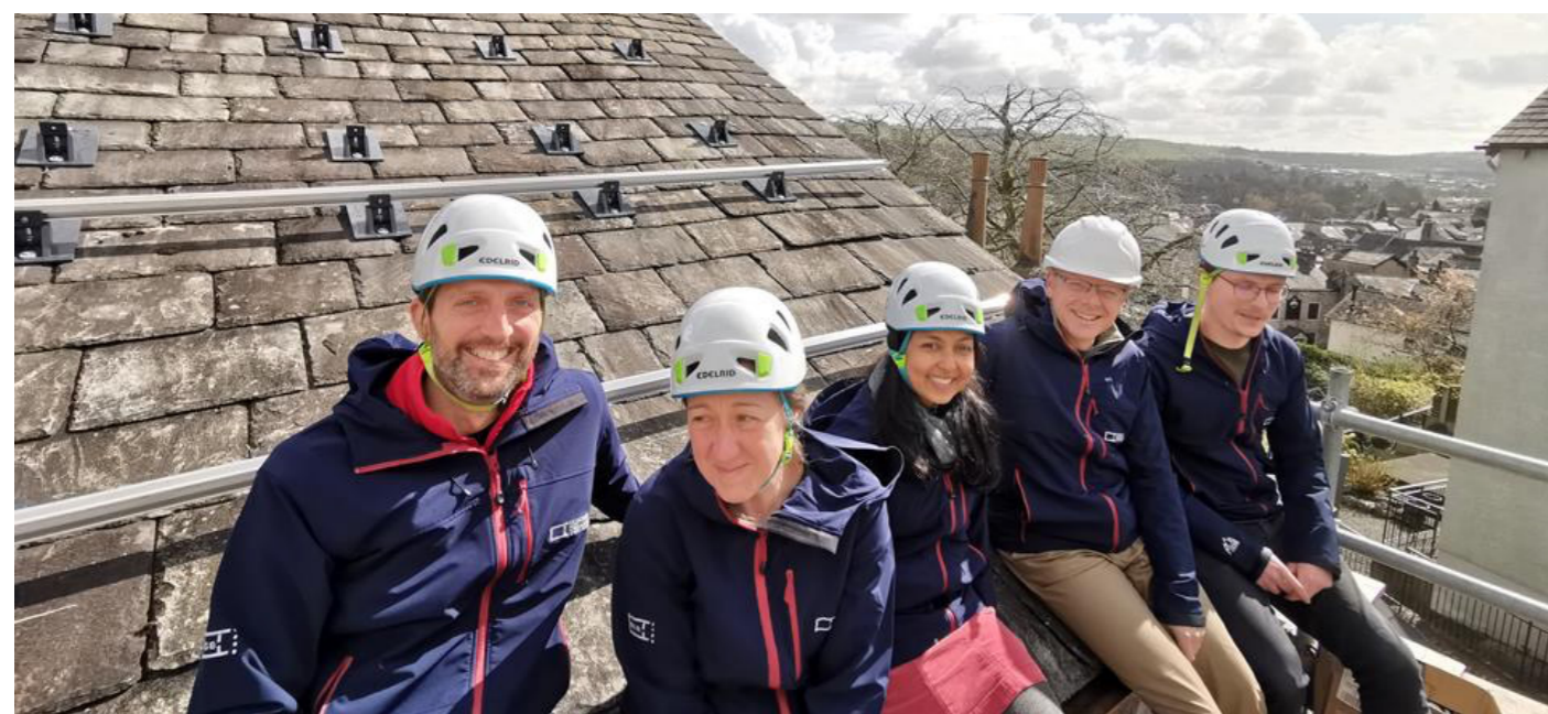
Preparation for the installation of solar panels at the headquarters of Crosby Grainger Architects (photo c/o Lake District Foundation)
