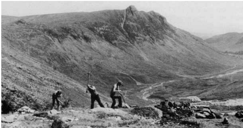
Path repair at Rossett Ghyll.
