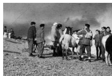
Rebuilding the Helvellyn shelter.
