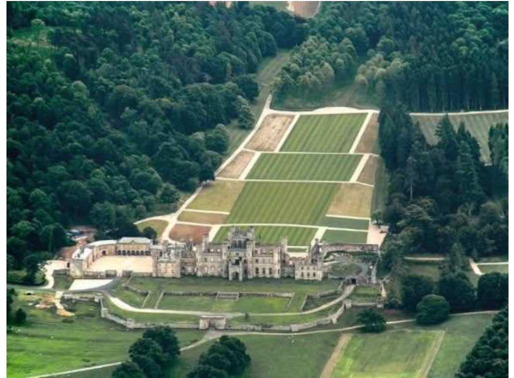
Figure 5.2 Lowther Castle post-restoration works
