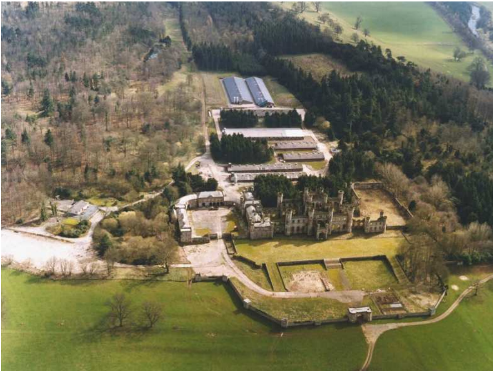
Figure 5.1 Lowther Castle pre-restoration works
