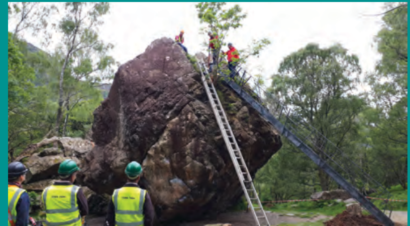
Above - 2018 work on the new access ladder.
