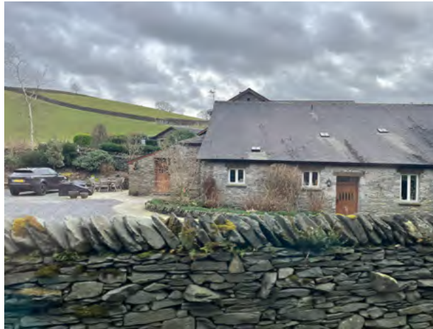
6.1.1 Farm buildings converted into residential accommodation
