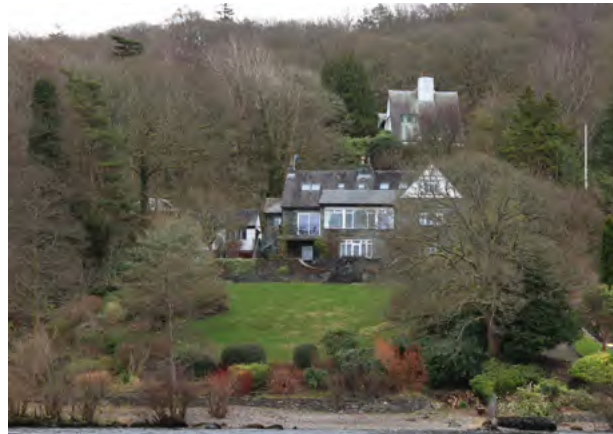
5.5.5 Terracing to 19 th century villa
