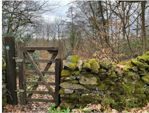
7.2.12 Dry stone wall boundary typical of the CA
