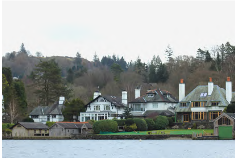
3.1.8 Residential buildings to eastern shore
