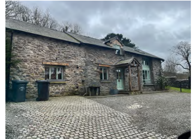
6.1.2 Single pile historic farm building
