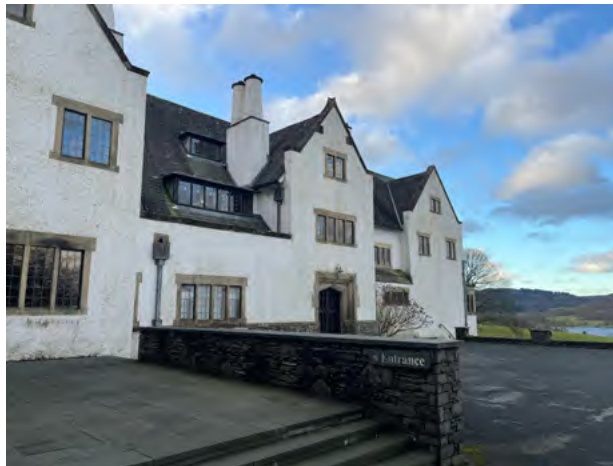
6.4.5 Blackwell from entrance courtyard
