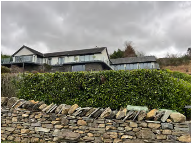
7.2.14 Suburban character resulting from hedging and walling
