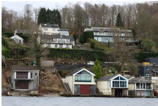
5.5.10 Lost landscaping to formerly open plots
