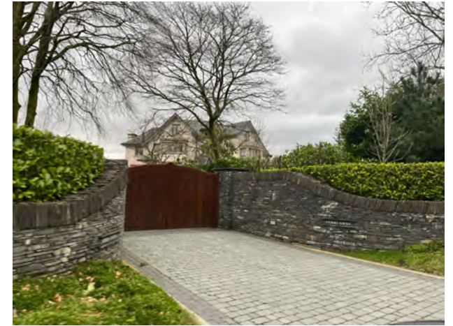
7.2.13 High boundary wall and gates to properties
