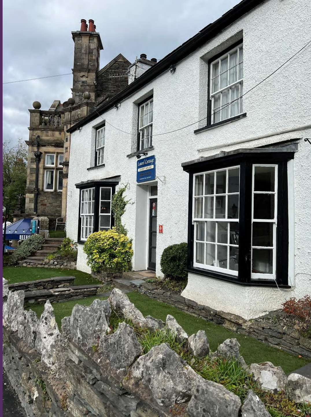
Front elevation of Laurel Cottage as seen from public views from the road
