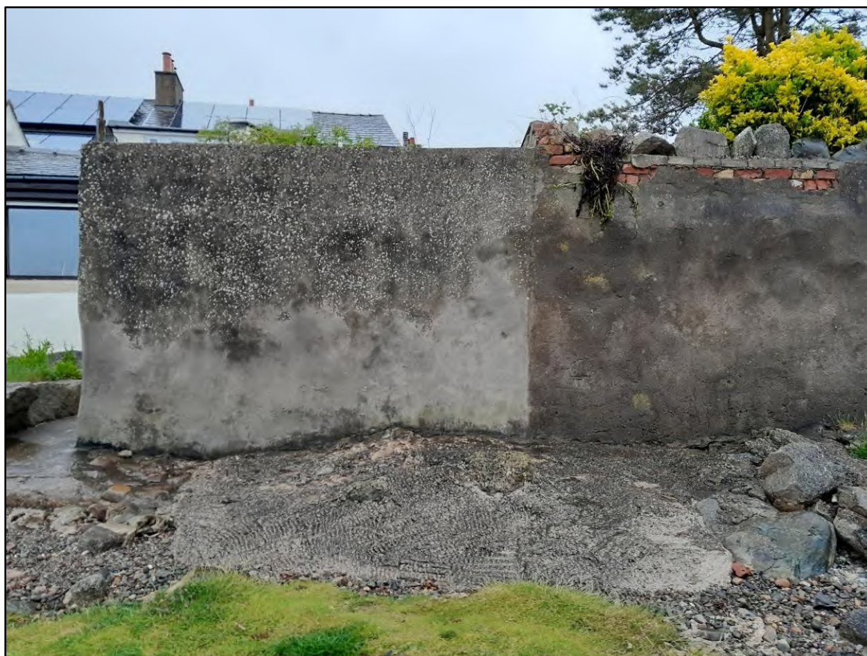
Item 43 – Photo taken during site visit June 2024 – although now rendered, the two different sections of seawall can be easily distinguished
