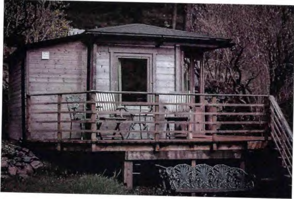
The Hut measures 4.25m X 3 m
