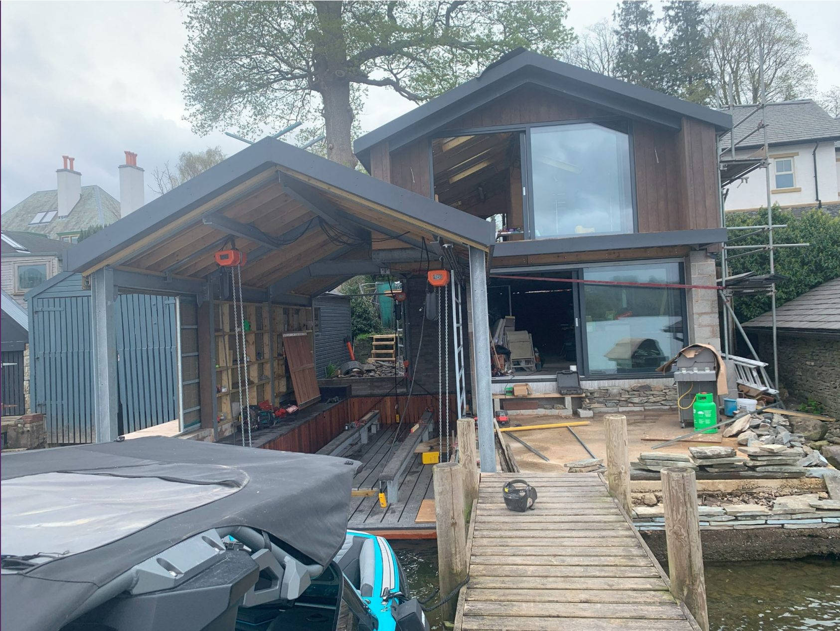
Photograph of West Elevation
