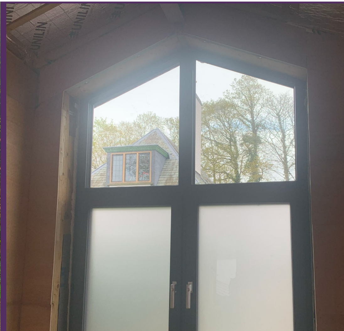
Photograph from window on east elevation looking towards Brunton
