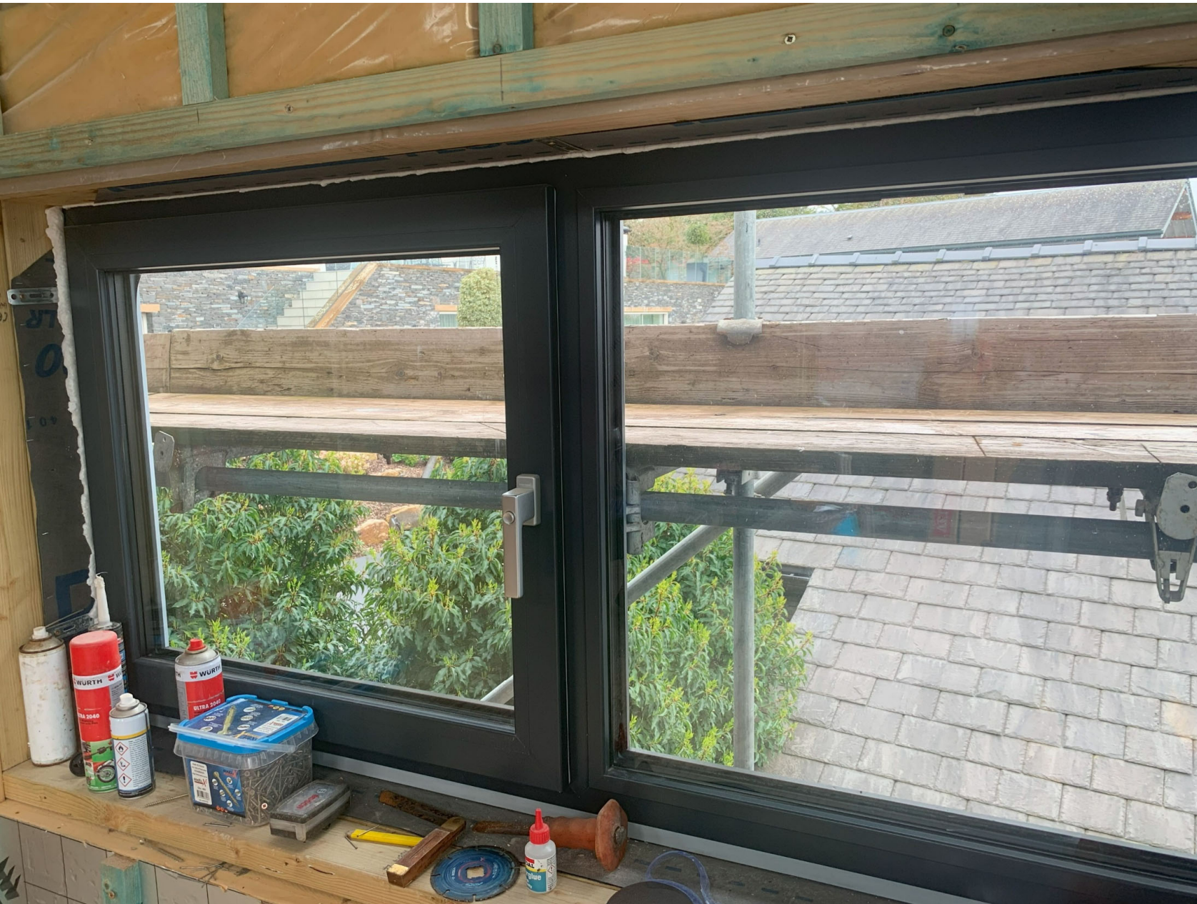
Photograph from window on the south elevation looking towards Storrs Holme
