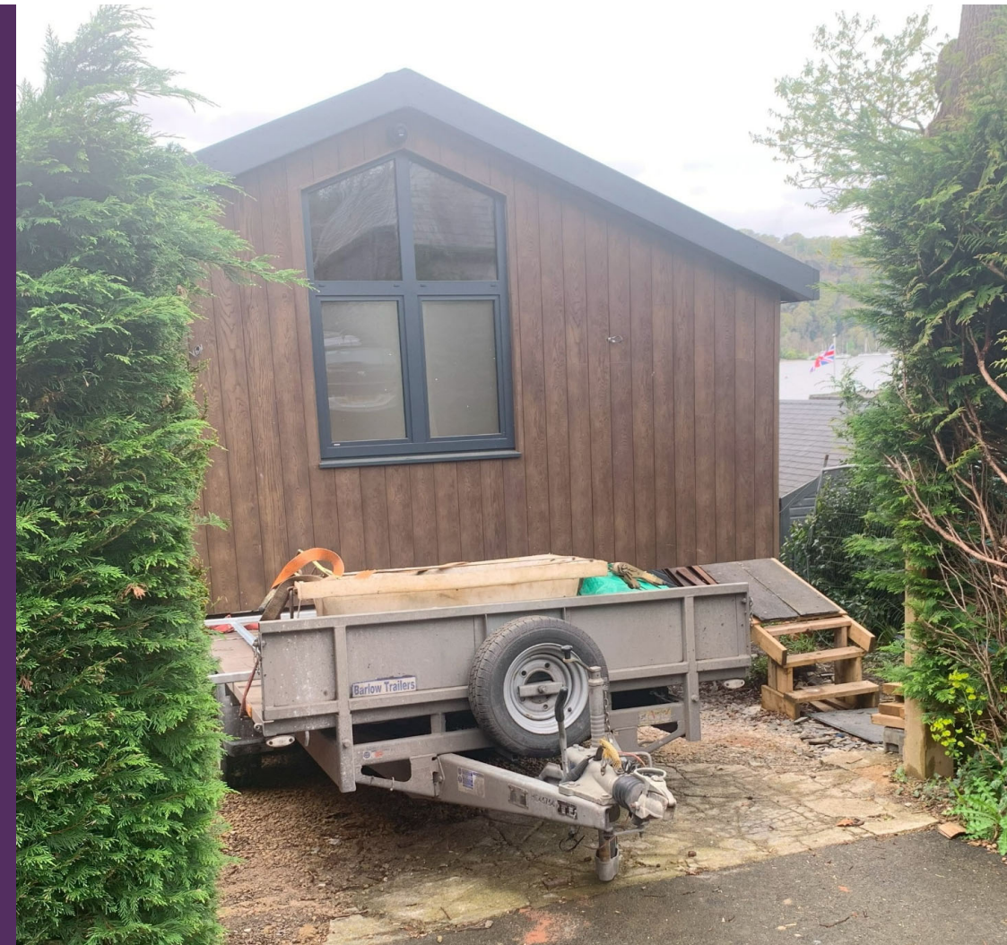
Photograph of east elevation
