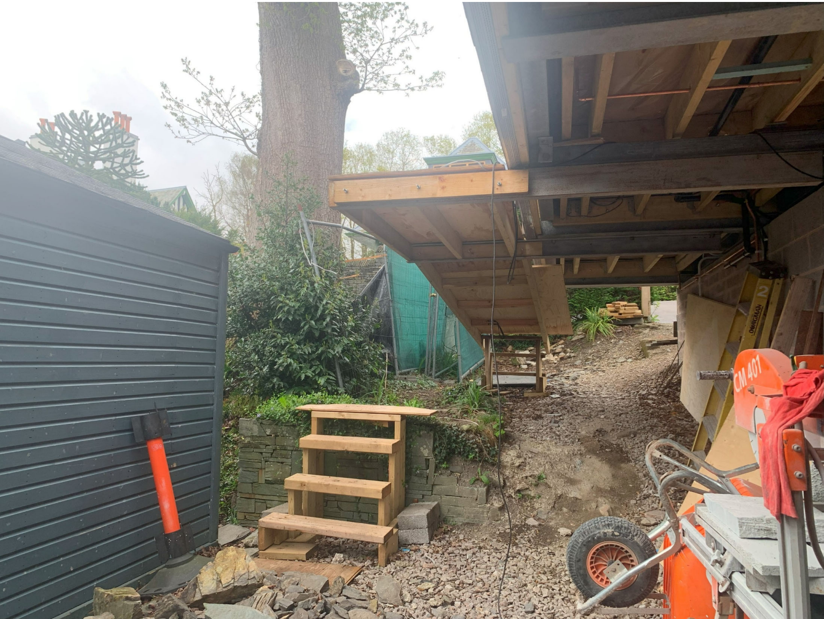
Photograph of area for new external stairs
