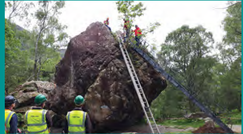
Above - 2018 work on the new access ladder.
