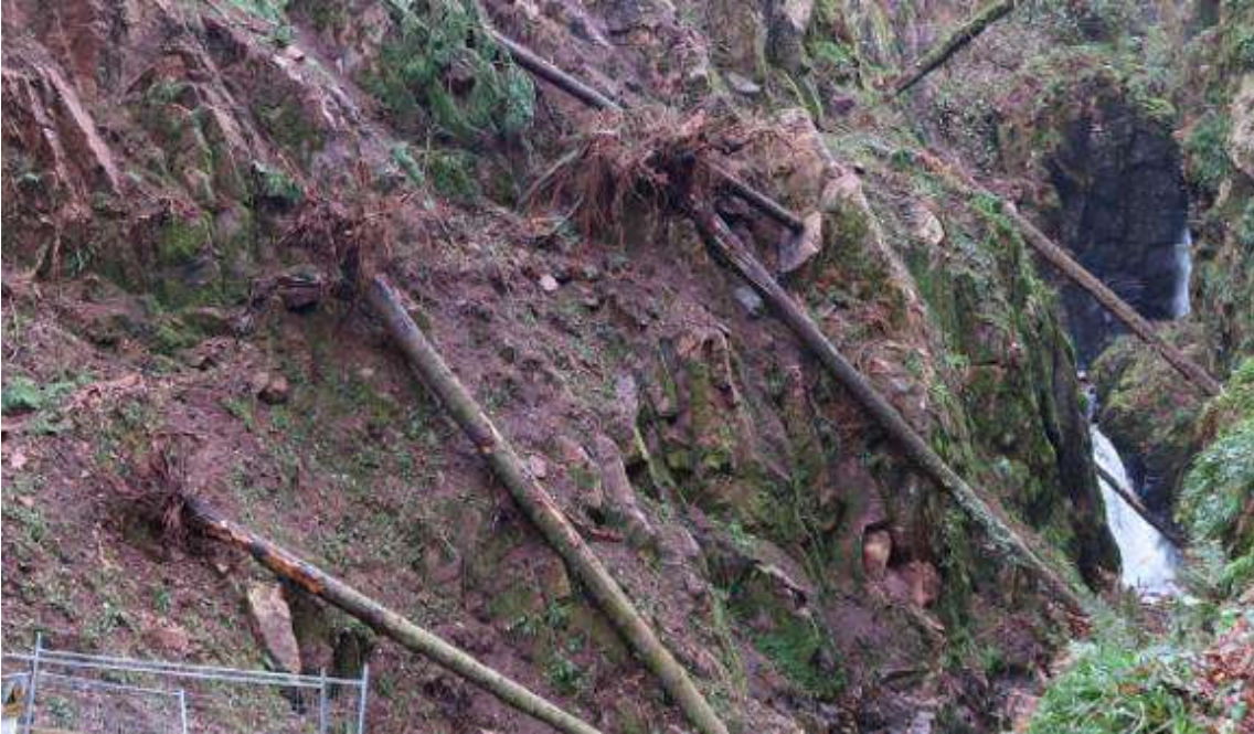
Photo 3 – Windblown trees felled by storm events, the upturning of the rootballs has further destabilised the surrounding rock contributing to the hazard. Where trees have fallen down this causes further scouring and destabilisation of the slope.
