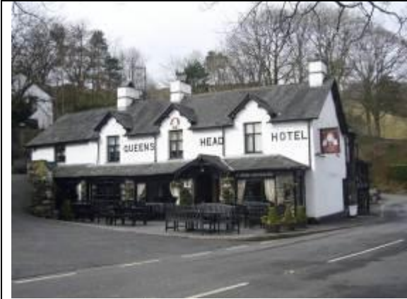
Fig. 47 The Queens Head has 17 th century origins but has been much restored, listed grade II. This façade is 19 th century.
