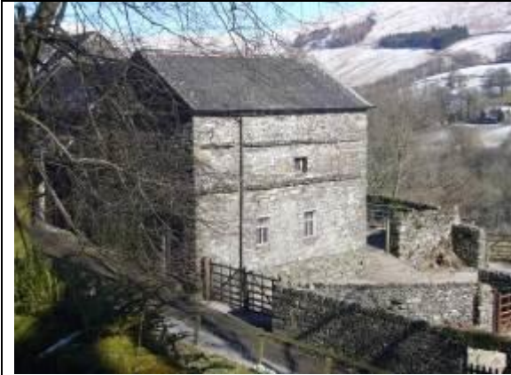
Fig. 17 One of the two projecting wings of the barn at Townend, listed grade II*.
