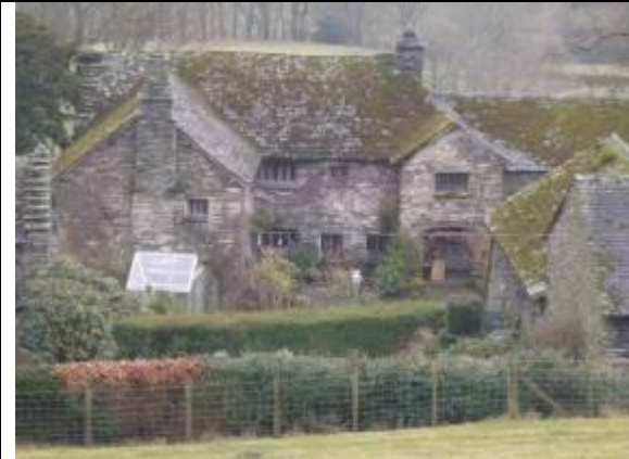
Fig. 39. Thwaite Farmhouse – once derelict it remains a most picturesque vernacular building of great rustic charm, listed grade II
