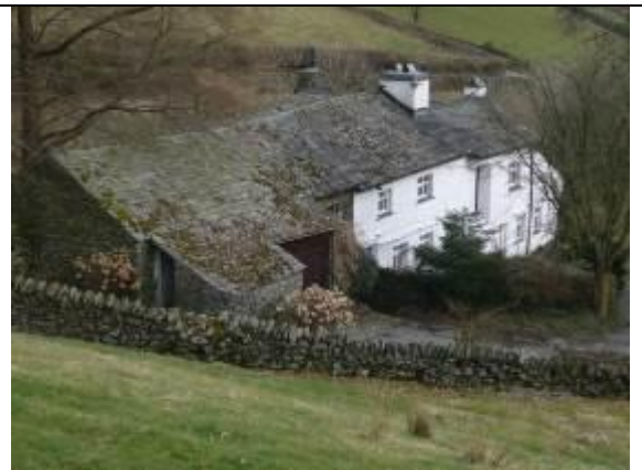
Fig. 6 Jownie Wife House, with a converted granary at the far end, nestles into the hillside.
