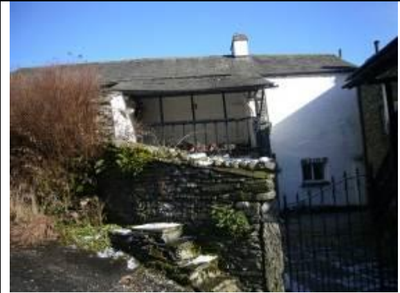
Fig. 9 A 'spinning gallery' at Yew Tree Cottage. It is unlikely that covered balconies like this were actually designed to shelter spinners.
