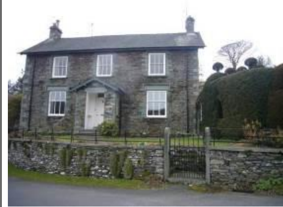
Fig. 41 Town End House is a 19 th century attachment to a 17 th century building. Quoins and window dressings are probably of imported limestone.
