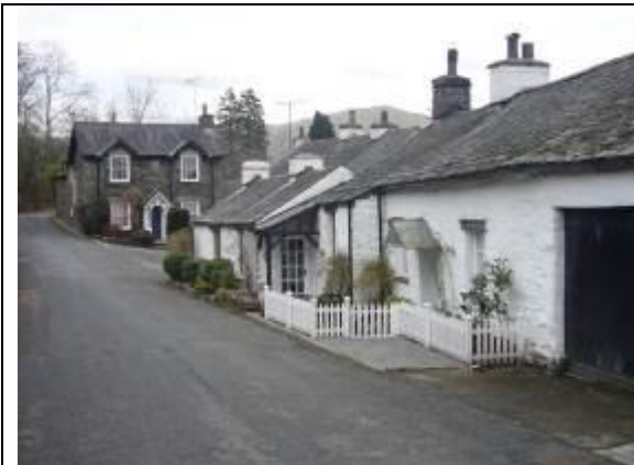
Fig. 33 The canopy at Longmire Yeat Cottage, in the foreground, is made of two projecting stone slates fixed above the front door.
