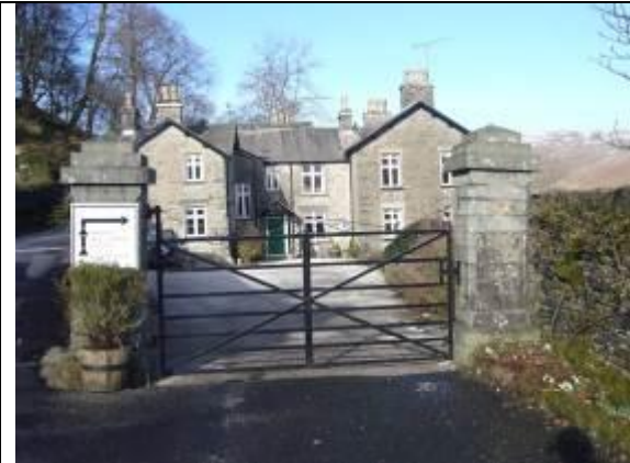
Fig. 23 Birkhead is a late 19 th century construction. Compare the chimney stacks with Troutbeck Hall (adjacent photo). Clay chimney pots are a Victorian introduction.
