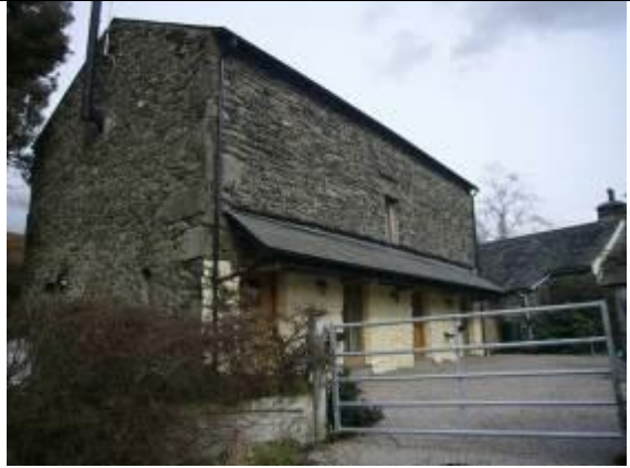
Fig. MP1 This former barn has been sensitively converted without additional openings and retaining original exposed stonework and vernacular detail.
