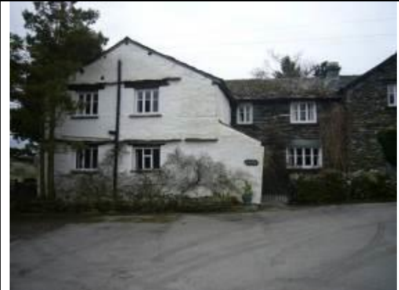
Fig. 21 Farmhouse at High Fold. Note the contrast between exposed stonework and render or limewash, a typical feature of the village.
