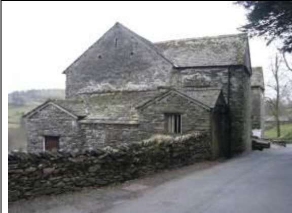
Fig. 1 The barn at Townend dates from the mid-17 th century and is listed grade II*.
