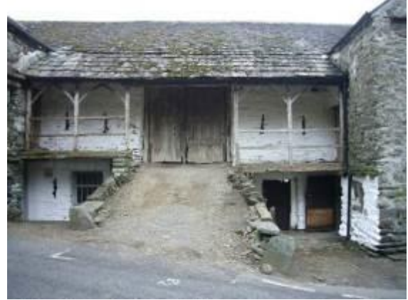
Fig. 42 Townend barn (1666, grade II*). The canopy over the ramped entrance to the upper barn has been extended as a gallery, giving covered access to the barn's two wings.
