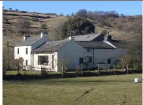
Fig. MP8 Large areas of glass in horizontal openings ('picture windows') are out of character with historic cottages.
