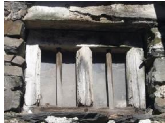
Fig. 45 Wooden mullioned window at Townend barn, possible re-used from a house.
