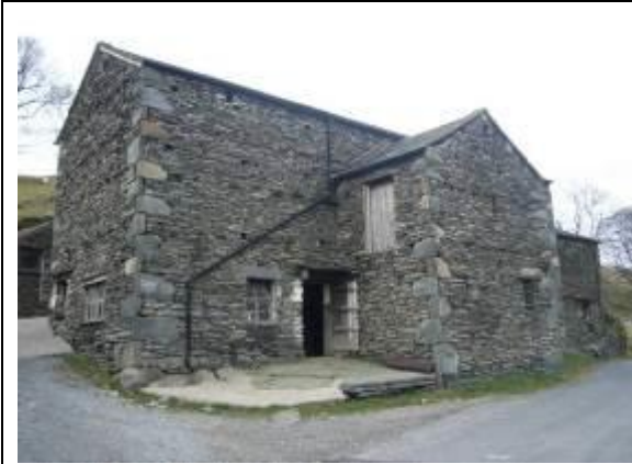
Fig. 25 A bank barn by Lanefoot Farm. The first floor door was used to load wagons. The upper storey is accessed from the rear (up the slope).
