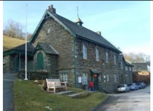
Fig. 2 The Institute is a Victorian addition to the village that now houses post office and shop.
