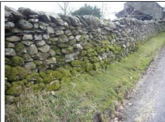
Fig. 5 Characteristic stone roadside wall with a narrow grass verge.
