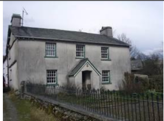
Fig. 28 This building in High Green dates from the 18 th century, listed grade II.
