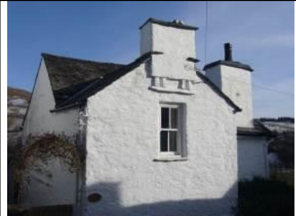
Fig. 37 Storeythwaite, listed grade II. Note how the chimney stack projects beyond the gable and there is a small window below.
