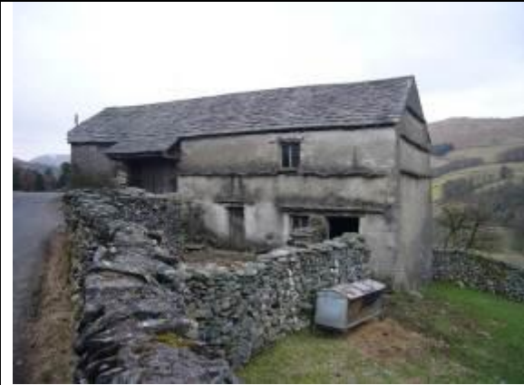
Fig. 19 Unlisted barn to the south of Matthew How dramatically situated overlooking the valley below.
