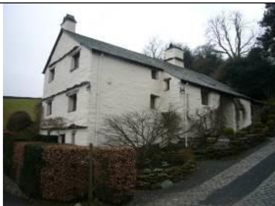
Fig 15 Town Foot is a 17 th century building. Note the small size of the windows and high ratio of solid to void, i.e. large area of walling and small window openings.
