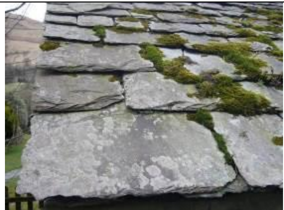
Fig. 34 Stone roof slates from a local quarry, laid in random widths.
