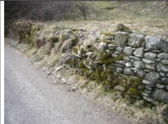
Fig. MP5 Loss of sections of walling or of capping stones detracts considerably from the character and appearance of the conservation area.
