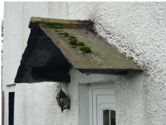
Fig 19: A rare example in Staveley of a simple slate-stone porch
