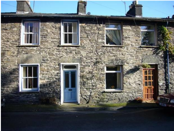
Identical cottages with original door and windows on the left and modern replacements on the right
