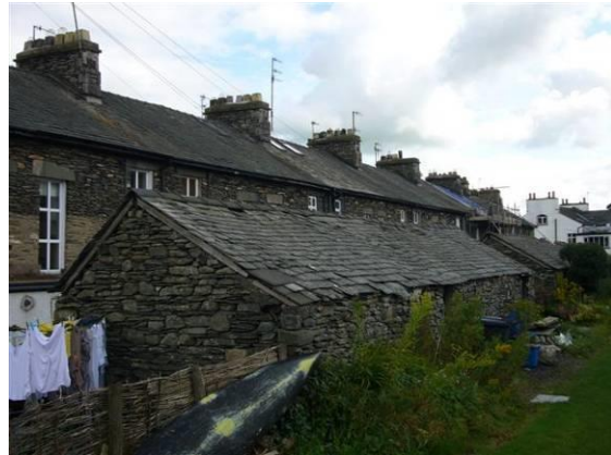
Fig 21: Original outhouses in Gowan Terrace
