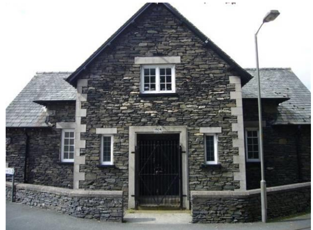
Fig 25: 'Dry-stone' construction used for the Village Hall
