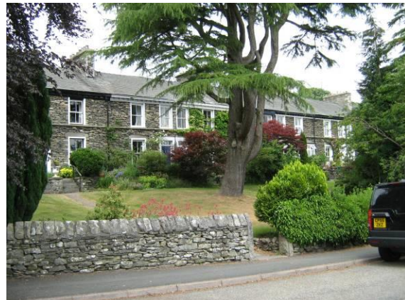
Fig 8: Danes Row – a fine Victorian terrace marking the westward entrance to the conservation area
