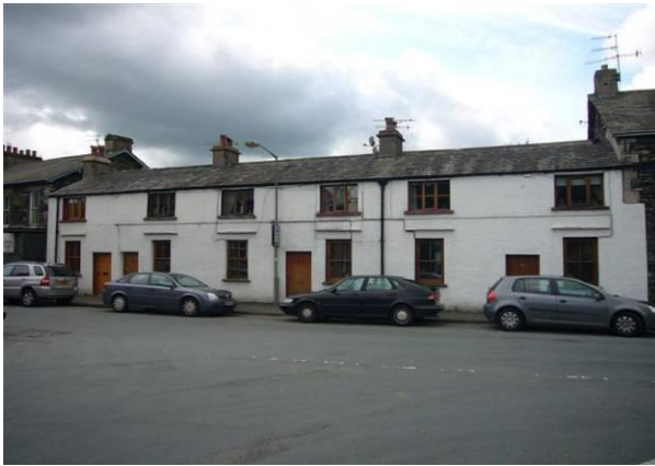
The use of stained door and window joinery and the alteration of door and window openings
