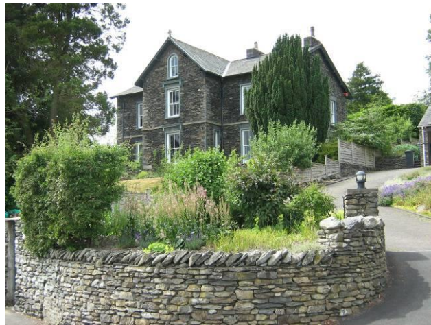
Fig 28: The Vicarage on Brow Lane – a significant unlisted building of historic character
