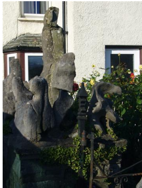
Fig. 15: Limestone pavement used as coping – a characterful if environmentally harmful Victorian fashion
