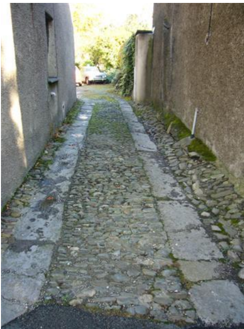
Fig 16: The cobbled yard to No. 65 Main Street.
