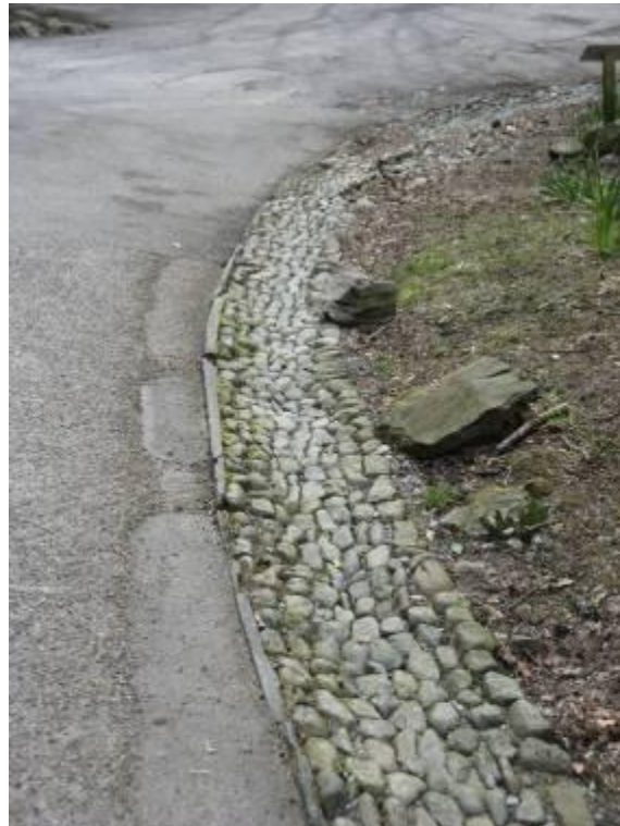
Fig. 12: Substantial stretches of historic cobbled floorscape survive, making an important contribution to the character of the village.
