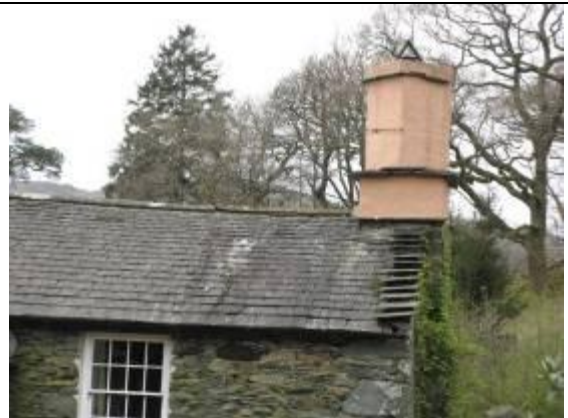
Vernacular features at Hart Head include the polygonal chimneystack and the stepped gables created from large slates.
