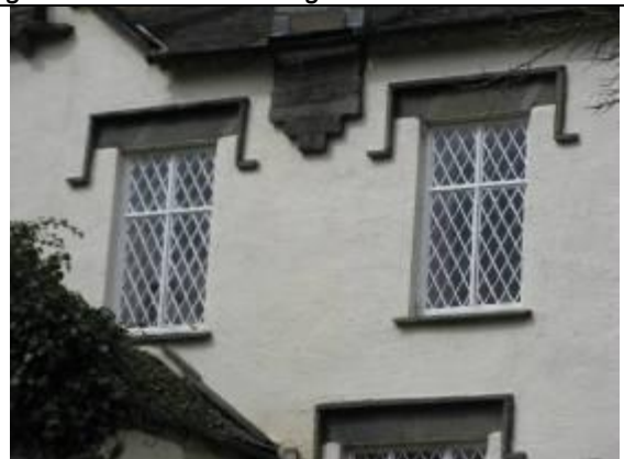
Undermount is a 19 th century fusion of vernacular and neo Tudor features and displays these attractive leaded lights.
