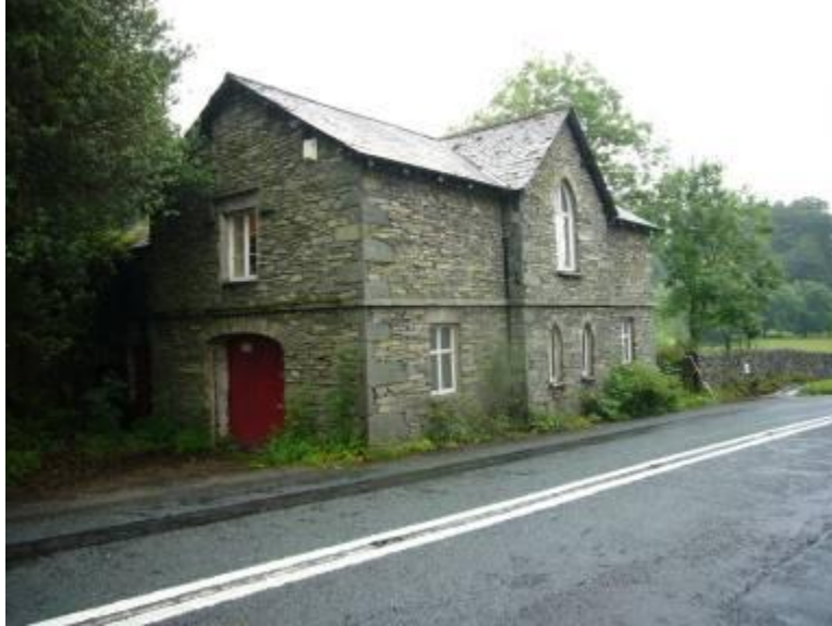
Fig. 9: Defining the south-eastern entrance to the village is the Rydal Institute, built like a Lakeland barn (note the large quoins made of slatestone set on edge) with an external staircase to the rear. Note too the park landscape beyond the Institute, the stone boundary wall, and the white milestone set into the wall.
