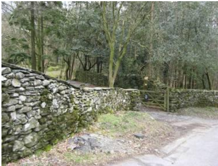
Fig. 11: Slatestone walls are the prevalent form of boundary treatment; here they have been unusually capped using Lake District slate.
