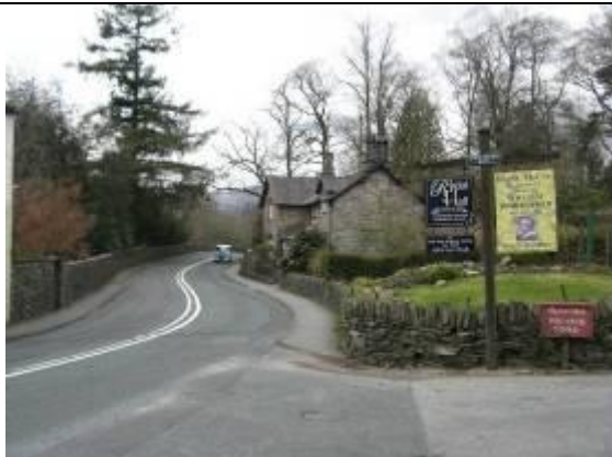
From the A591, the old turnpike road, there are views through the conservation area including to nos. 1-2 Rydal Cottages.
