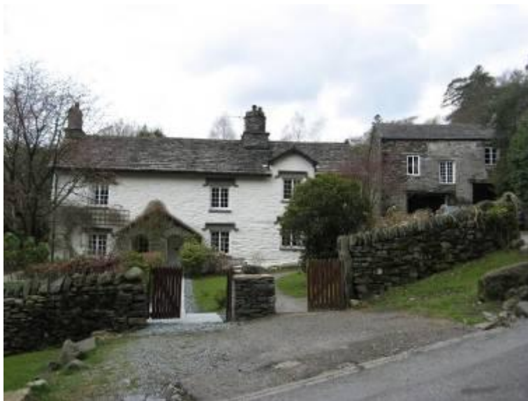
Fig. 13: Mount Cottages are a good example of vernacular building in Rydal, with distinctive circular chimneystacks and slatestone drip moulds.
