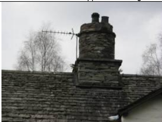
A large circular chimneystack at Mount Cottages.
