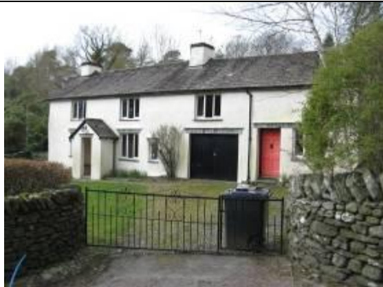
The insertion of this modern garage door in a historic building has partially eroded the character of the building.
