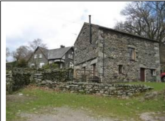
The converted barn at Hart Head displays features such as the ground-floor entrance to the cow house and the upper winnowing door.
