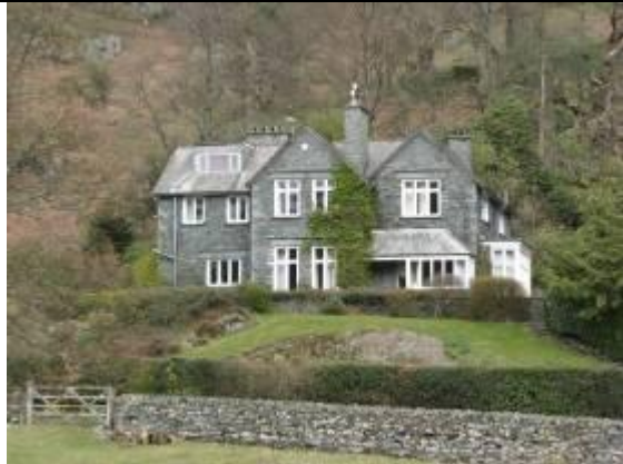
Alterations to historic buildings, such as the insertion of a box dormer, can threaten the historic character of an important building.
