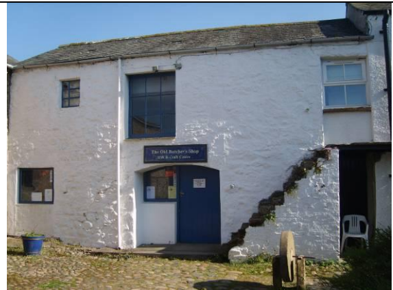
Fig 26 Former agricultural building to the rear of Main Street.
