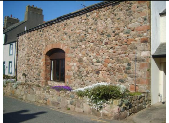
Fig 36 Former agricultural building now a dwelling in Main Street.
