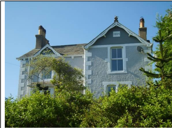
Fig 21 Springfield (1884) overlooks the railway junction.
