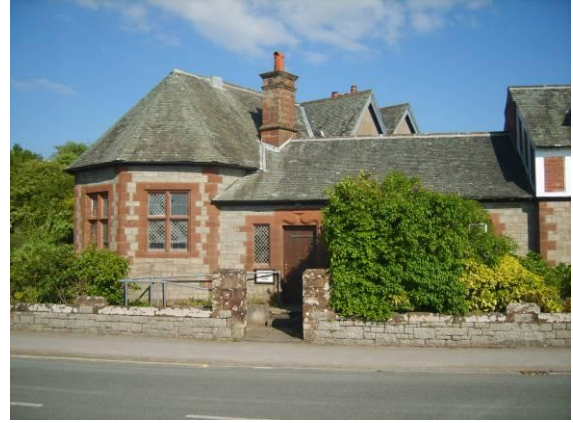
Fig 16 Former school and police station, Main Street.
