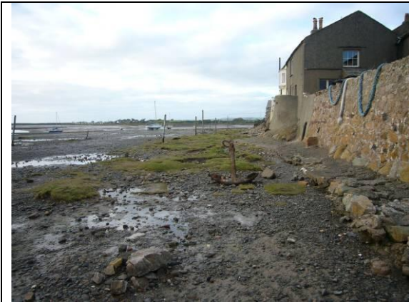
Fig 9 The west side of Main Street directly abuts the estuary.
