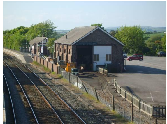
Fig 22 Former goods shed (c.1873) of the Furness Railway.
