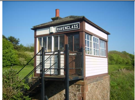
Fig 8 Signal box at Ravenglass Station.
