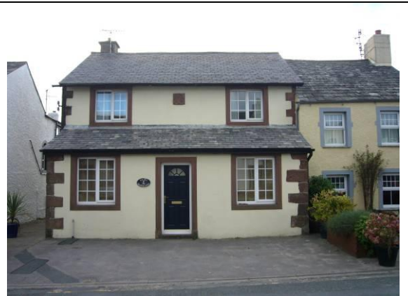
Fig MP2 The forecourt of this property has been designated entirely for parking.
