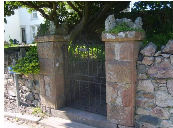
Fig MP3 Stone walls and gate piers add to the area's historic interest.
