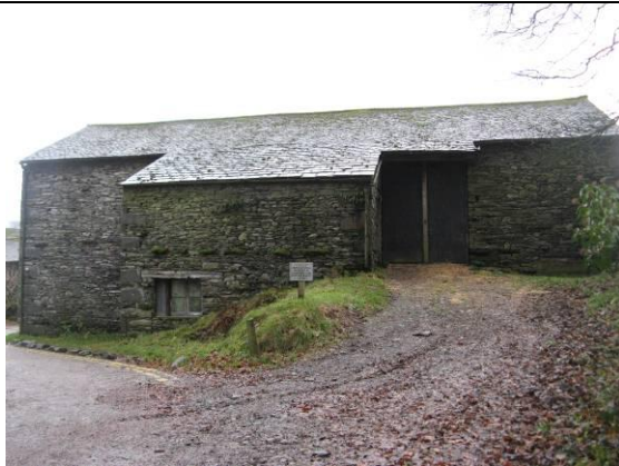
The bank barn (Saw Mill) features a ramped entrance up to the upper level.
