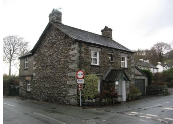
Anvil House is constructed from coursed slatestone.
