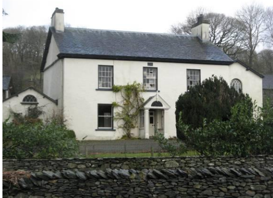
Tower Bank House is an early 19 th century parallel to the earlier vernacular cottages in the village.
