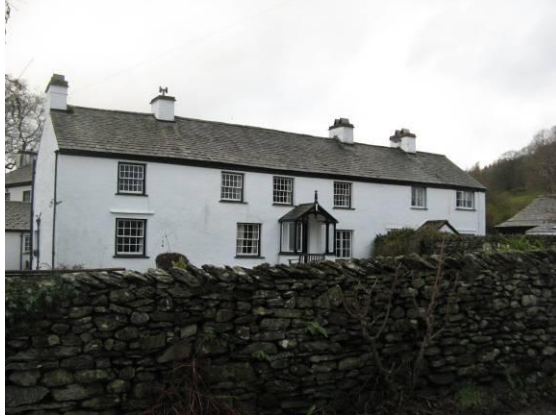
The 18 th century High Greengate features distinctive multi-paned timber sliding sash windows.
