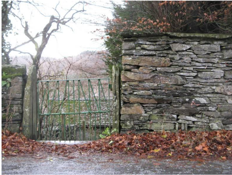
Fig. 9: Slatestone boundary walls are a distinctive feature of the conservation area.
