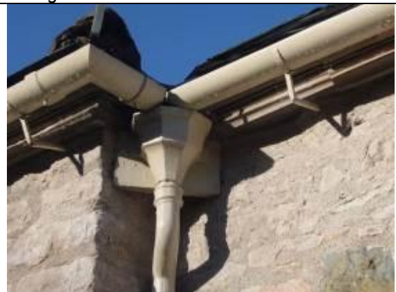
Fig. 12 Rainwater goods are cast iron painted in a uniform colour throughout.
