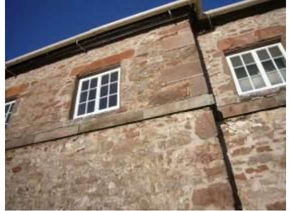
Fig. 32 Buildings are in a good state of repair.
