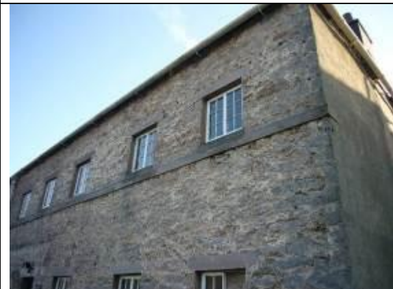
Fig. 11 The external stonework of this house in the western court retains traces of limewash.
