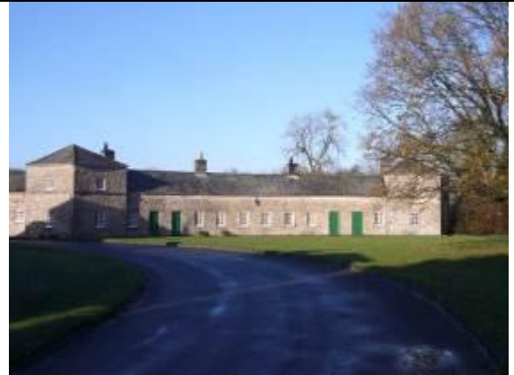
Fig. 20 First view of the circus on arrival from Hackthorpe, to the east.
