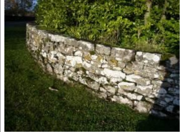
Fig. 31 The conservation area is characterised by stone boundary walls.
