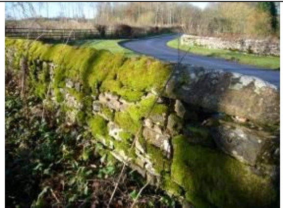
Fig. 8 Stone boundary walls are a feature of the conservation area. This one is topped with triangular coping stones.
