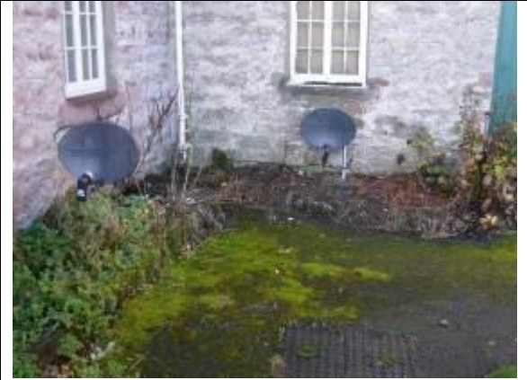
Fig. MP2 Satellite dishes in the western court.
