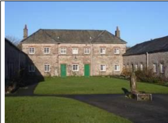
Fig. 21 The side ranges in the central court are single storey.
