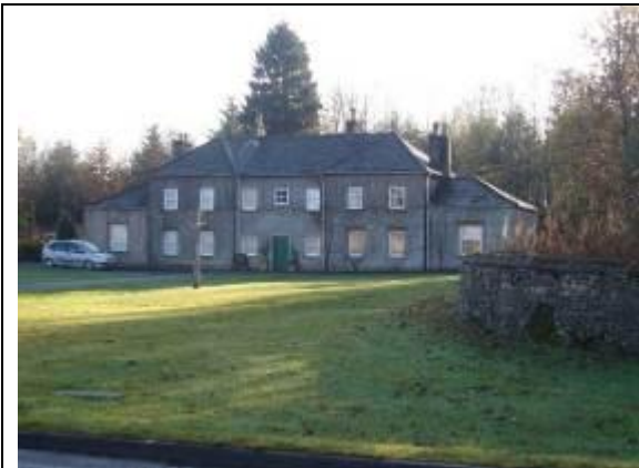
Fig. 3 Keepers House was altered in the 19 th century. Although it has kept its original form, the stonework has been rendered and the window openings enlarged.
