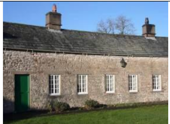
Fig. 4 Only two quadrants of a planned circus are standing. It is possible that two other quadrants of cottages were demolished in the early 19 th century.
