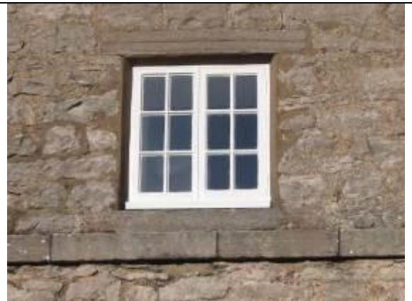
Fig. 6 Small-paned casement windows are the norm. The stone string course is one of the village's few architectural adornments.
