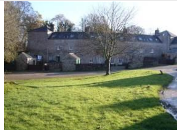
Fig. 27 Rear of the circus' north-west quadrant of cottages is, surprisingly, two storeys in height.
