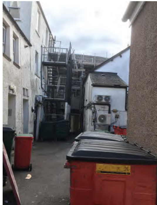
13.56 and 13.57 Wheelie bins and cars can block passageways, impede access for pedestrians, and are an unsightly introduction to the market place.
