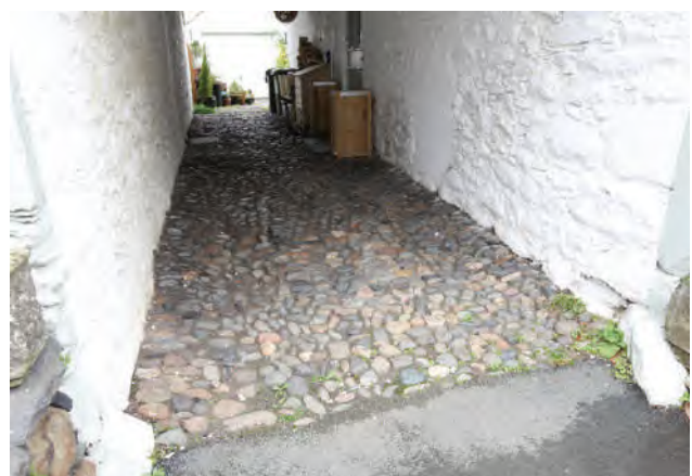
8.3 - Washed river pebbles from the Greta, laid to form a traditional cartway between private houses
