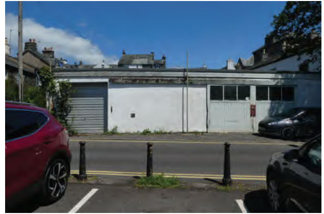
13.13 Modern commercial garages facing the central car park
