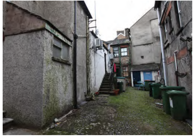
13.55 Private Yard off Paraffin Alley - original cobbled surfaces, and a largely forgotten space
