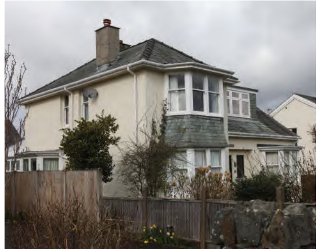
7.21 Hipped roof with slate hanging to projecting bays, roughcast and sash windows
