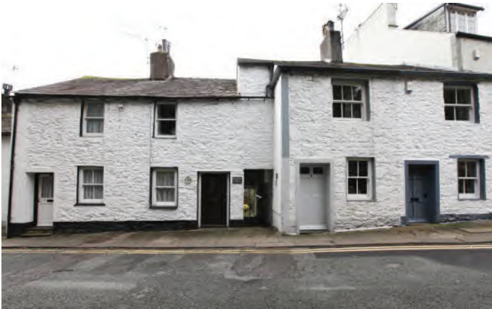
8.6 - 'The Plosh' - limewash is applied in multiple layers over the rubble stone, unifying the various phases
