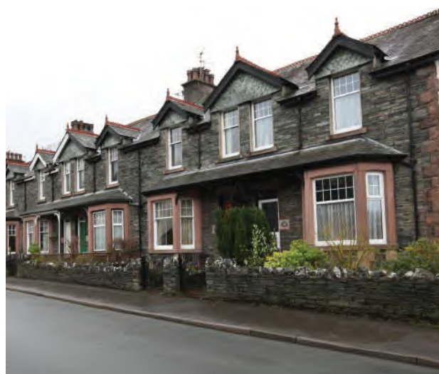
8.61 - typical late Victorian residential terrace on Blencathra Street
