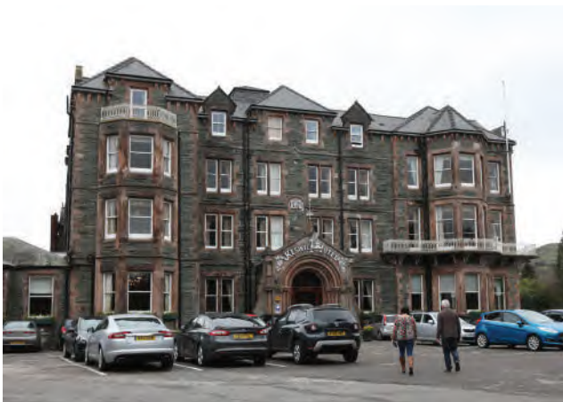
7.10 View of the large Keswick Hotel from the forecourt which is shared with the station, with an ornate porch emphasising the entrance.
