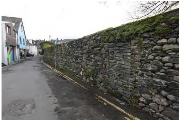
6.16 Gretaside - striking Borrowdale and dolerite boundary enclosure, removes views of car parking, and separates the industrial core from the town centre enhancing its distinct identity.
