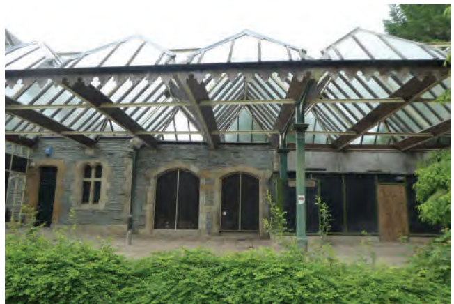
7.13 The dramatic, canopied glazed station platform is now part-absorbed within the hotel.
