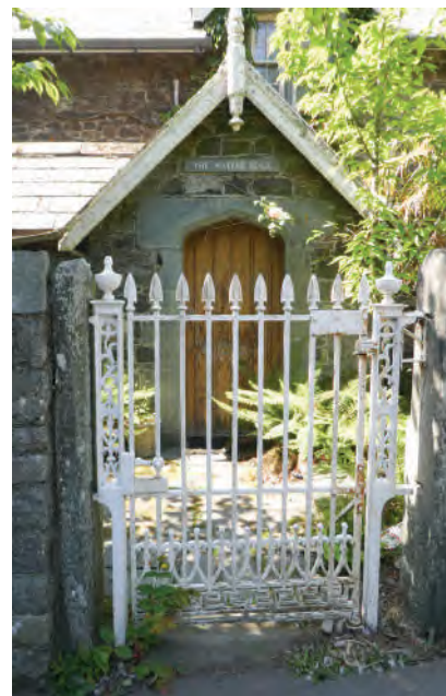
8.18 - 1840s cast-iron gate to The Water's Edge
