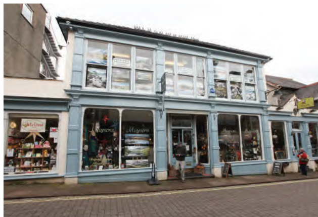
8.53 - Two-storey cast-iron shopfront - former Henry Mayson's Photographic Studio
