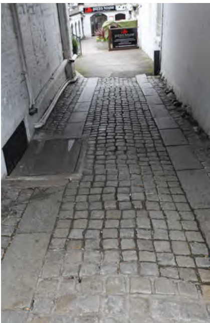
13.40 Threlkeld granite setts and flush kerbs - King's Arms Yard.
