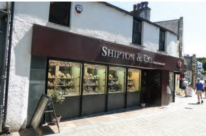
13.36 A fascia which is out of scale and disproportionately large for the small host building.
