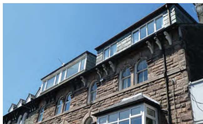
13.4 The dormers at Lake Road (right) were not recorded in the 1991 photographic survey, which covered only residential properties.
