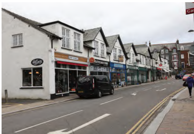
6.5 Nos. 3-19 Bank Street
