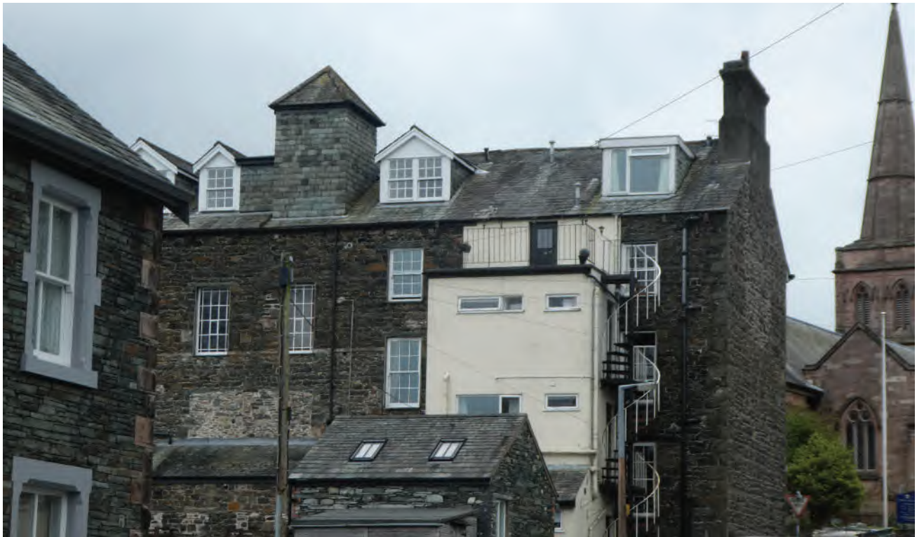
The harmful effect of flat-roofed rear extensions on prominent public views
