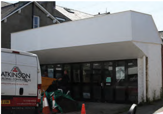
13.21 Inappropriate development within the Victorian terraces. Redevelopment is desirable.
