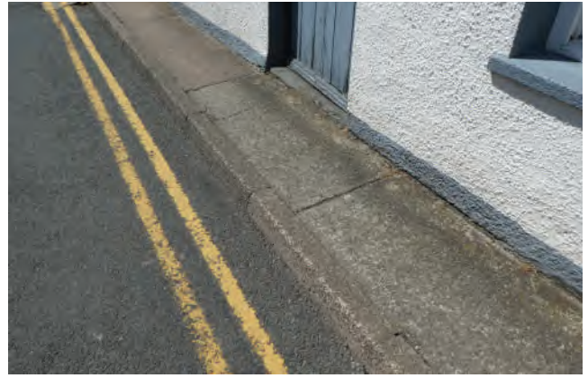
13.44 'Threlkeld' concrete flags and kerbs on Derwent Street.
