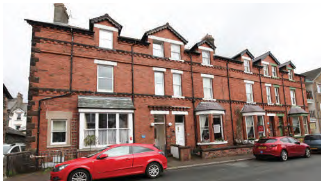
6.26 Rare use of red brick, with gabled dormers, bargeboards, bays and moulded terracotta details.
