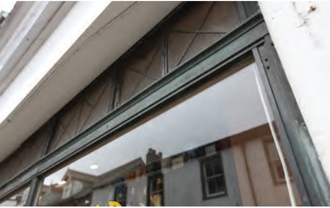
13.32 Original bronze shopfront with clerestory glazing to Premier at 5 St. John's Street.
