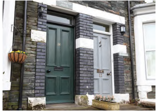
8.63 - Unusual details of blue brick dressings
