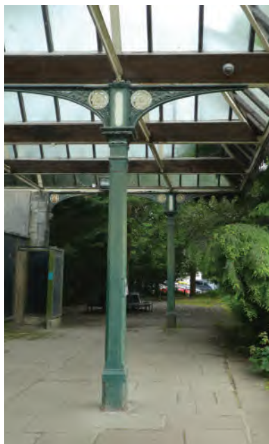
8.17 - Cast-iron post and spandrels to the station canopy.
