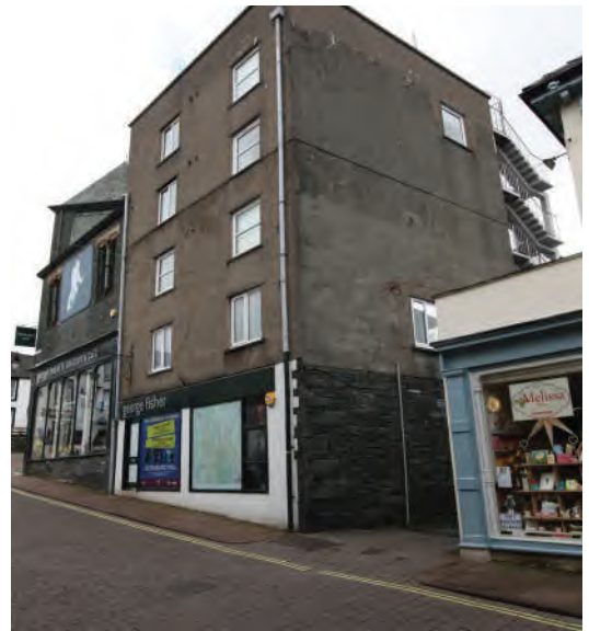
13.20 Inappropriate massing and flat-roofed development at Lake Road.
