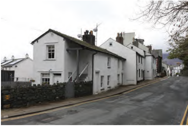
6.7 The Plosh, Borrowdale Road. The staggered row of painted and rendered cottages creates a visually interesting and welcoming entrance into the town from the south
