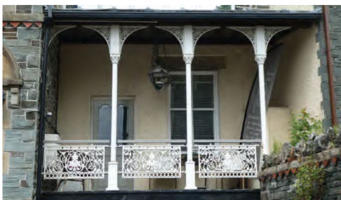
8.19 - Cast-iron panels, posts and spandrels used for a balcony on Station Road
