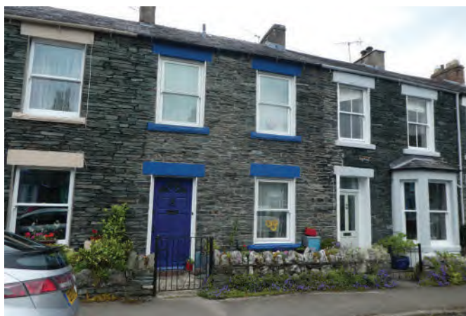
11.1 Re-pointing is seldom necessary with Lakeland slate, which is laid deliberately to shed rainwater.
