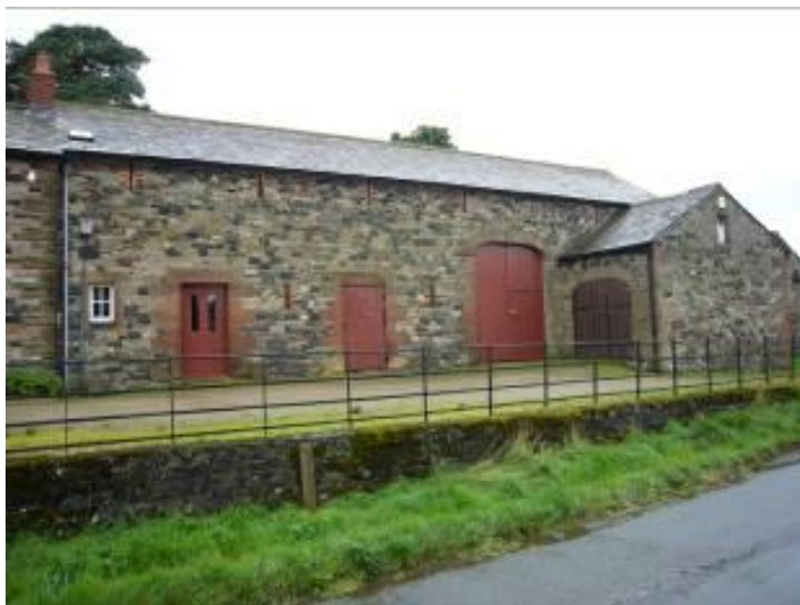
Fig. 23: Howbeck Farm barns: one of Hesketh's 'Significant Unlisted Buildings' and a superb example of this building type
