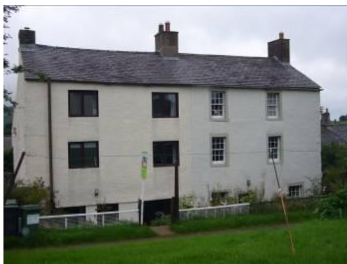
Fig 25: Compare the treatment of the two halves of the same building, one with original window openings and sash windows, the other with enlarged window openings and modern single pane windows
