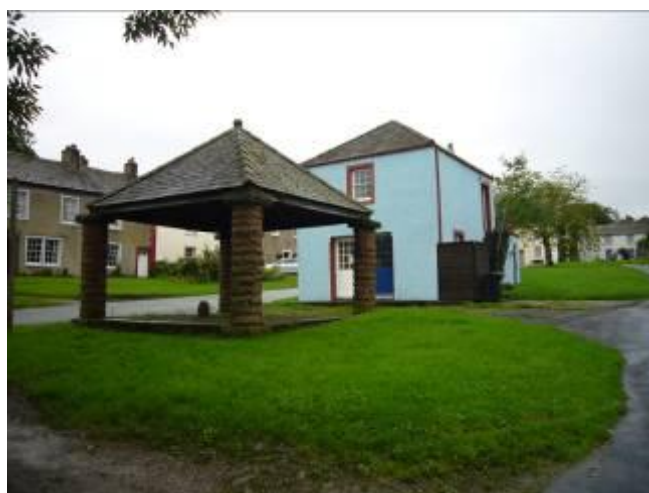
Fig. 4: The Market Cross and Coach House to the rear (Grade II listed - described in the listing as a "Moot Hall and coach house")
