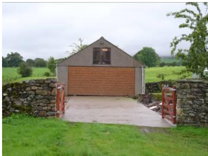
Fig 28 Highly visible outbuildings
