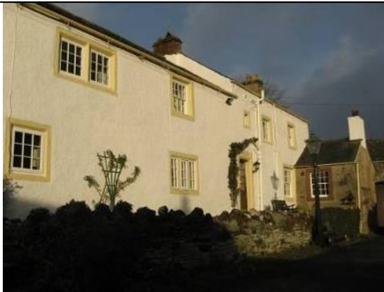
Square windows at Town End House display a mixture of flat mullions and chamfered reveals.
