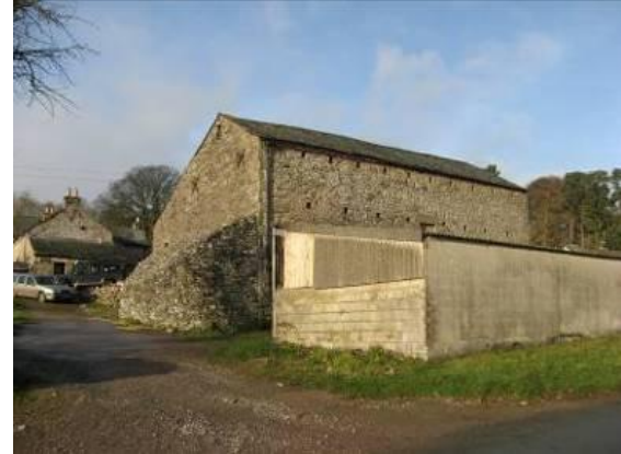
Modern farm buildings detract from the setting of historic agricultural structures.
