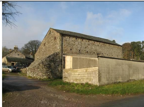
A large barn at Low Side Farm displays square ventilation holes.
