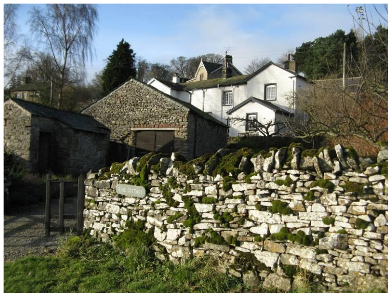
Fig. 11: Limestone rubble boundary walls are a distinctive feature of the conservation area.
