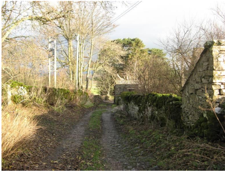
Fig.7: The back lane forming the north-western boundary of the conservation area is overgrown and impassible in places.
