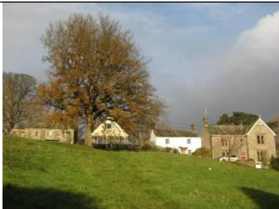
The view westwards up the slope of the village green is terminated by the row of buildings on the upper lane. The mature oak tree is an important local landmark.
