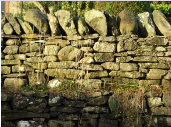
Limestone rubble walls are the predominant boundary treatment for fields.
