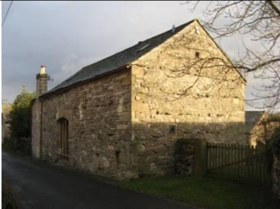
The barn at Low Side Farm has been converted but retains the former cartshed entrance. It also provides a good example of the use of 'throughstones'.
