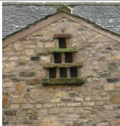
Nesting boxes in a gable wall of a barn at Low Side Farm.
