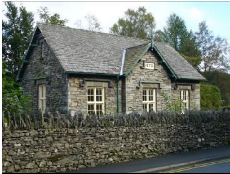
Fig. 3: The old school of 1873 shows the use of slate-stone with hidden mortar for the walls and green-grey Lakeland slate for the roof, while the boundary wall is a mix of water-eroded rubble from field clearance and quarried stone.
