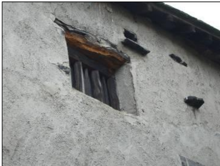
Fig 17: Post-medieval timber-mullioned window in Wordsworth Street
