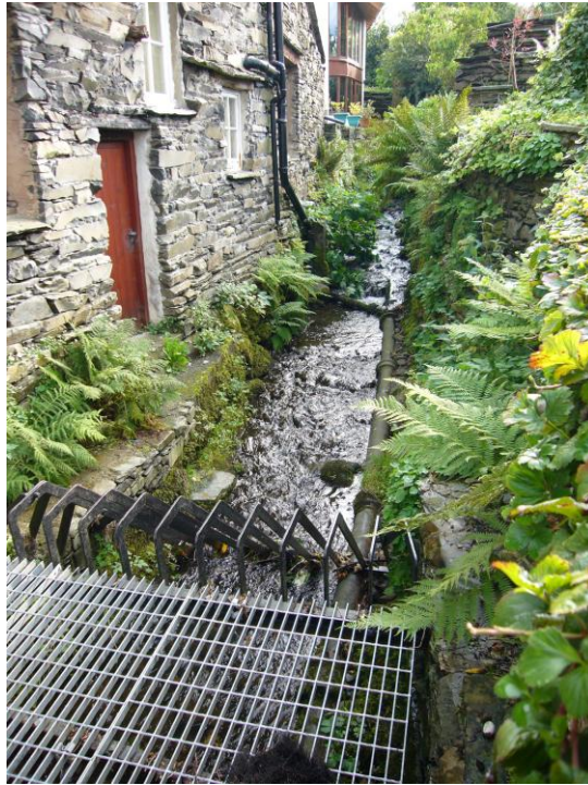
Fig.10: Black Beck which runs beneath the village within a culvert
