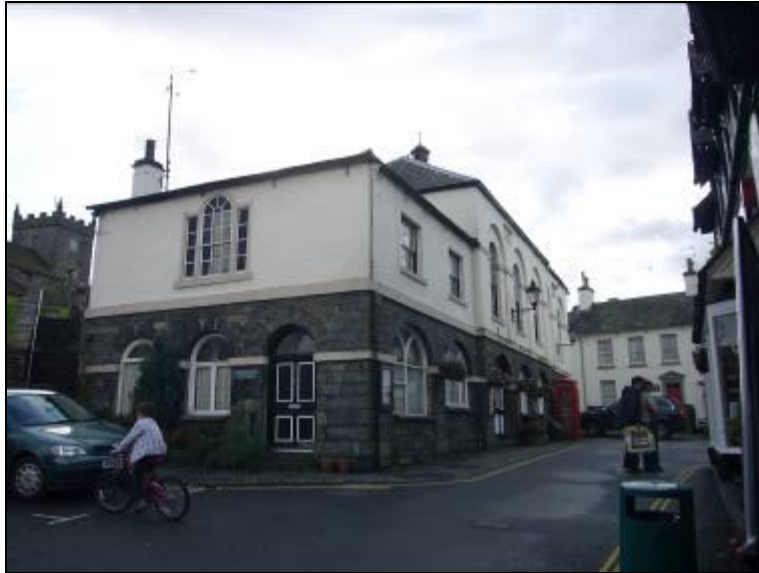
Fig. 5: The Town Hall was built in 1790, enlarged in 1887 and housed a market (The Shambles) in the arches below the meeting room, now filled in.
