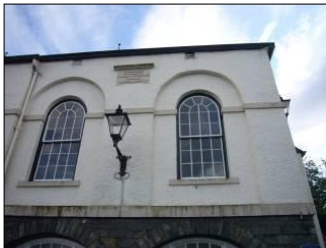
Fig 16: Wall mounted lanterns on the front of the Town Hall.
