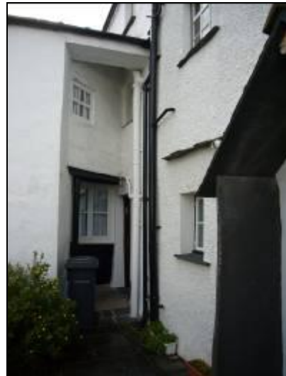
Varnished replacement windows.
