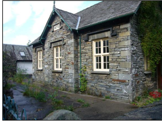
The Old School House is a vacant unlisted building. Permission exists for its conversion.
