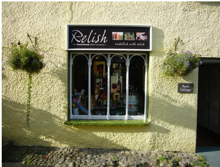
Fig. 24: Retaining traditional shopfronts and paving and sensitive new signage
