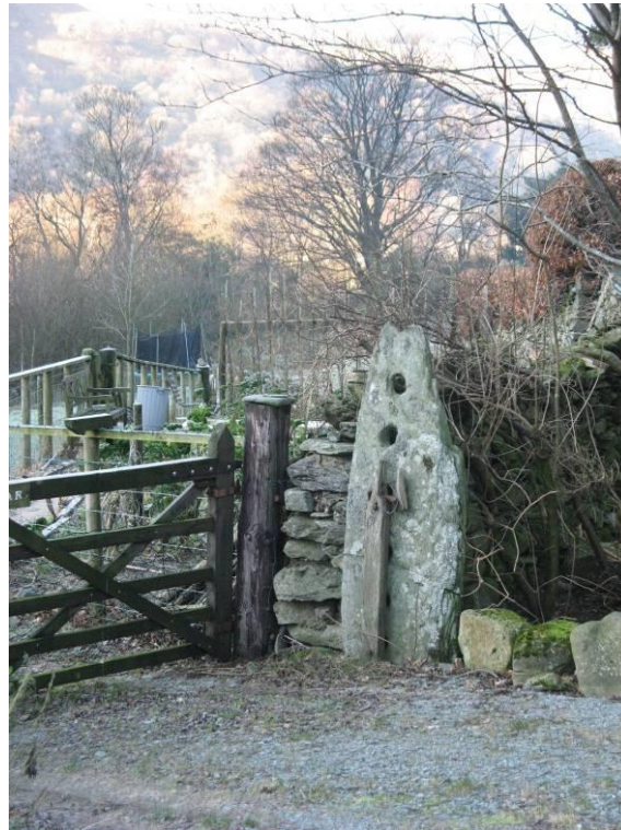
Fig. 12: Slate gateposts are a common feature. Note the holes for insertion of timber rails
