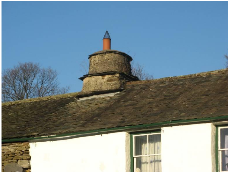
Fig. 13: Circular chimneystacks are a vernacular feature found on some of the historic buildings, such as this one at How Green.
