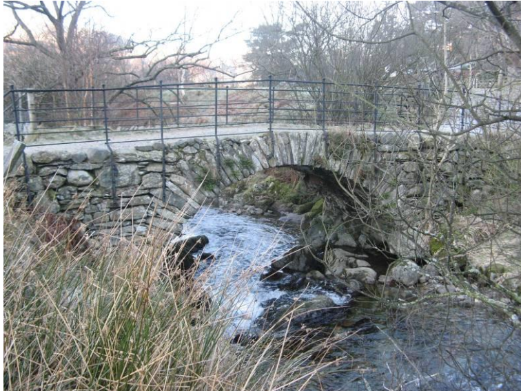
Fig. 15: Walker Bridge is a 17 th century pack horse bridge.
