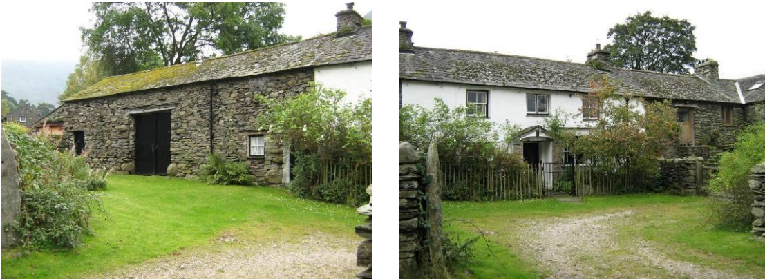
Fig. 5 Low House (right) a former farmhouse and its two barns (right and left) share a single roof.
