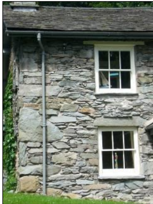
Fig. 13: Thimble Hall demonstrates some typical Lakeland vernacular features, such as massive quoins (here set alternately vertical and horizontal), deeply overhanging eaves and slate-stones of various sizes and colours set in broadly horizontal courses, with triple-paned sash windows.
