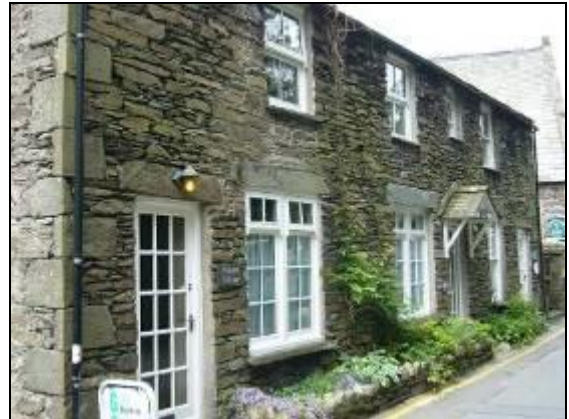
Replacement doors and non-traditional top-hung sash windows.
