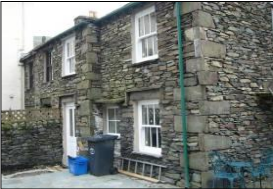
Massive quoins, hidden mortar, the use of blue- and purple-hued slate-stones, slate drip moulds and triple sashes are all defining characteristics of the local building style.
