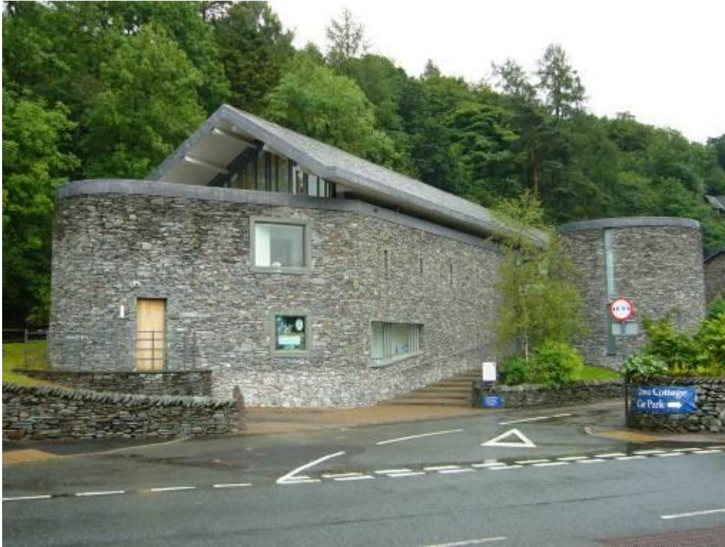
Fig. 2: The Jerwood Centre (2005) is an award-winning building using traditional stone and slate in a strikingly contemporary design.
