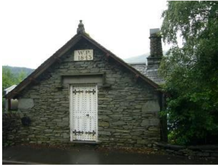
Fig. 13: The boathouse at the entrance to the village perfectly encapsulates the features of Lakeland vernacular with its overhanging eaves, columnar chimney and slate stone walls and roof.
