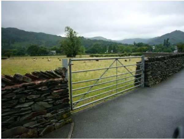
This tubular steel gate is harsh industrial intrusion into a timeless landscape, as is the pink cement based mortar used to finish what is otherwise a good Lakeland wall.
