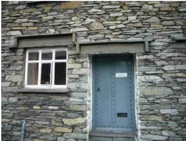
Many different window styles are found in Town End: here an opening central casement between two fixed panes.
