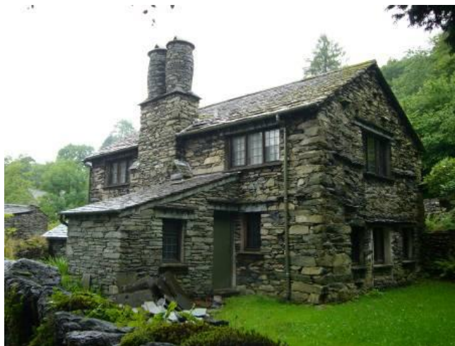
Fig. 14 Old Sykeside was formerly a barn and was converted in the 1930s when new windows, boiler house and chimneys were added.
