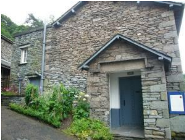
1 Town End nestles against the slope of the hillside, with its typical Lakeland quoins and drip moulds and its heavily studded door.
