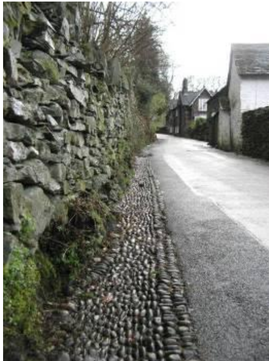
Fig. 1: Cobbles laid in traditional Lakeland style line the edge of the rural lane (a former packhorse track) that runs up to White Moss Common
