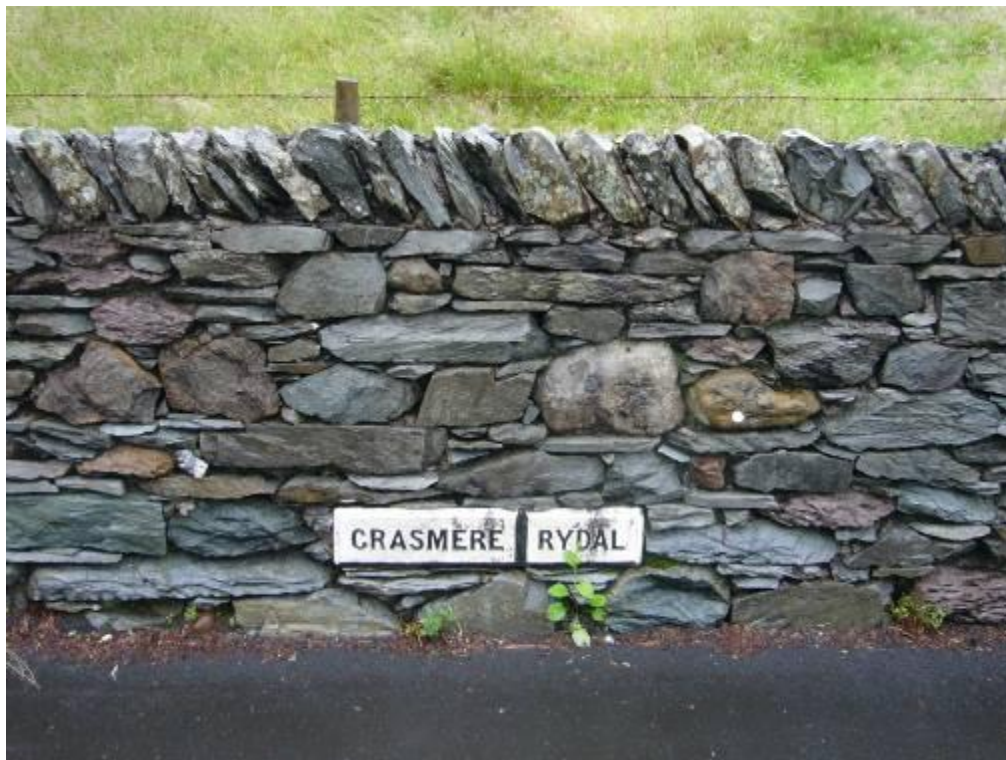
Fig. 11: The distinctive boundary walls of the conservation area are formed from randomly laid courses of slate stone with cappingstones set on edge. Here too the inset plaque marks the boundary of the parishes of Grasmere and Grasmere Town End.
