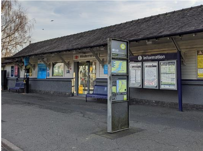
Windermere Train Station entrance with existing wayfinding signage.
