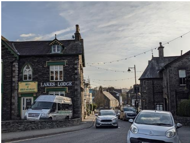
Grade II listed No 1 High Street.
