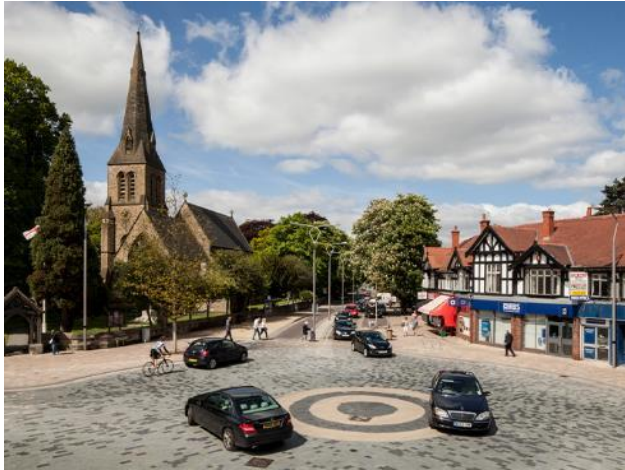
Poyton, Cheshire - Roundabout with material changes to reduce speeding and creating an attractive streetscene.
