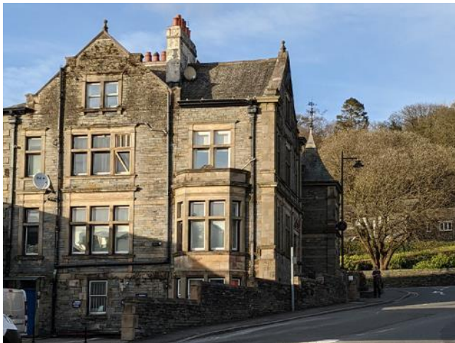
Building of Special Character along High Street.
