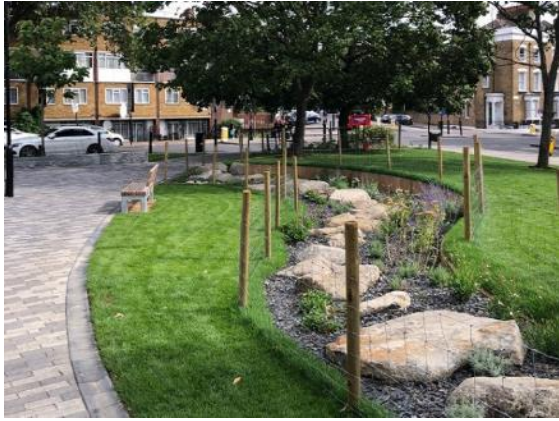
Canbury Station, London - suds incorporated into public realm.
