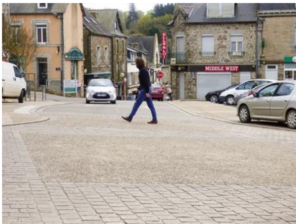
A change in surface materials creates a clear pedestrian priority environment in Brittany, France.
