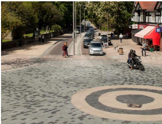
Material changes to the roundabout.
