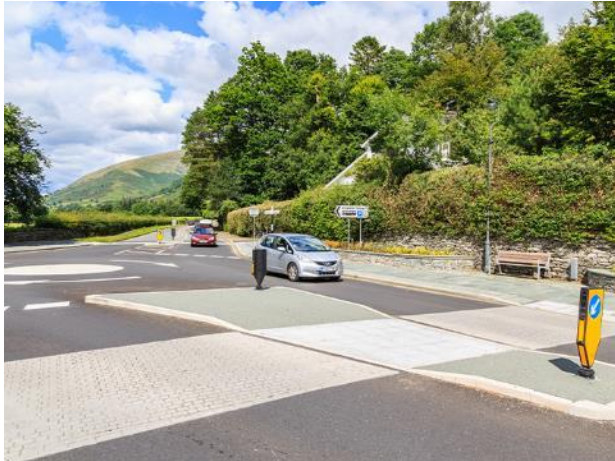
Pedestrian crossings in Grasmere. (© Capita Real Estate And Infrastructure; Cumbria County Council)
