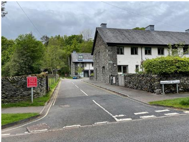
Grasmere, Broadgate Orchard affordable housing access - stone and slate boundary walls with paths for pedestrians.
