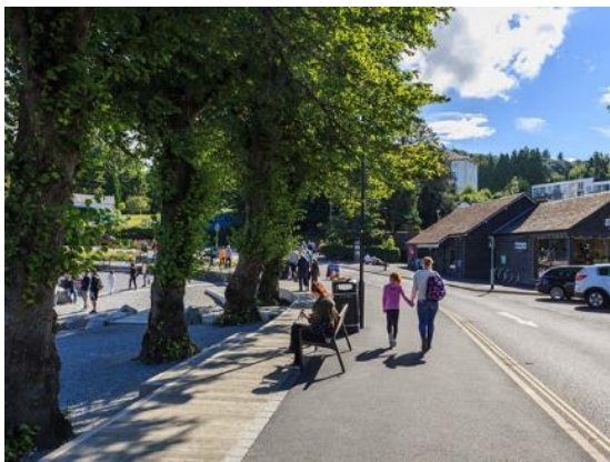
Attractive, well-defined street - The Glebe, Bowness Bay (© : Capita Real Estate and Infrastructure; Cumbria County Council)
