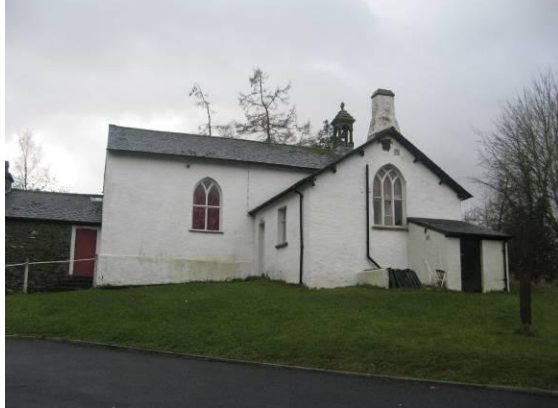
There are clear views of The Braithwaite Hall across the open car park which lies to the fore.
