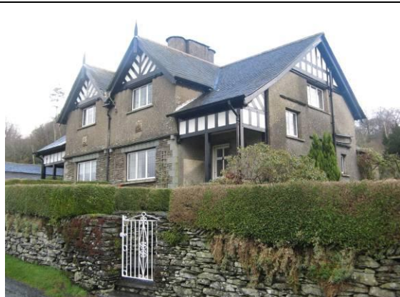
Glenside and Bishop Howe are a pair of cottages dated 1902. The cottages utilise both vernacular and Arts and Crafts detailing.
