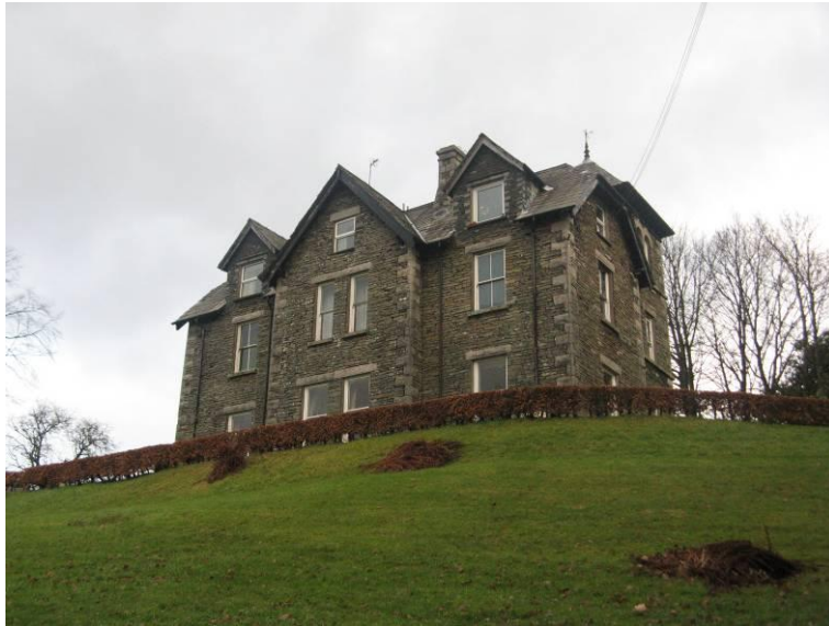
Fig 4: The Vicarage lies immediately outside of the northern limit of the conservation area. It is recommended that it is included within the conservation area, being of architectural and historic significance in association with Far Sawrey.
