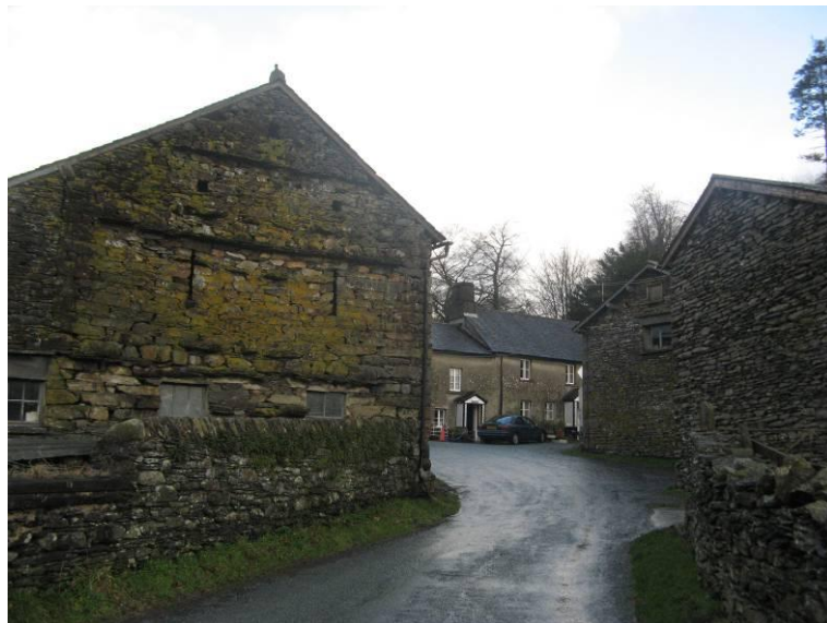
Fig. 14: View northwards to Sawrey Fold Farmhouse, past the associated farmbuildings.
