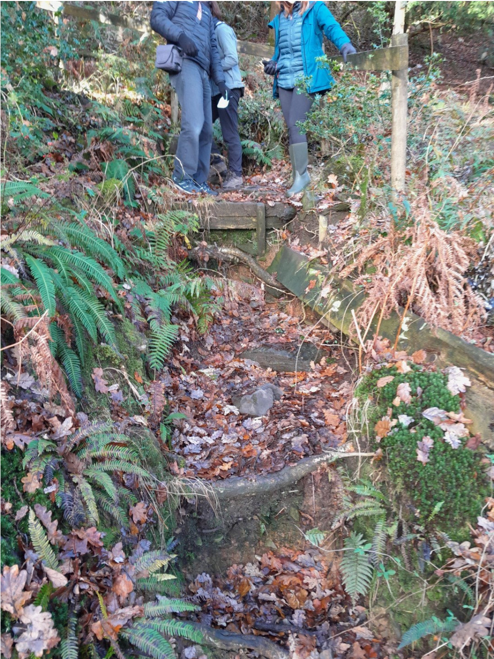
An example of some of the old steps that have now been replaced (the top step is higher than it looks)
