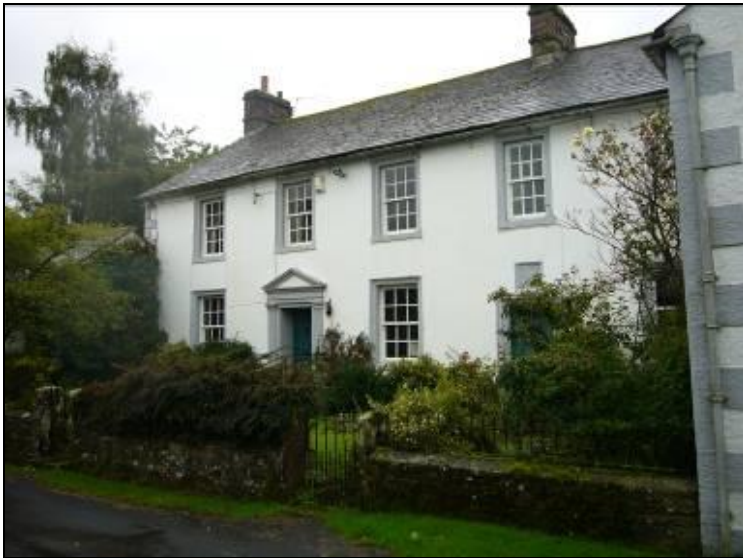
Fig 24: Bridge End House
