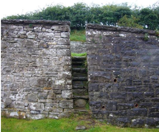
Fig 16: 1928 terrace retaining wall and steps near Hodden Croft Cottages
