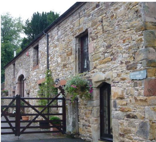
Fig 23 The use of red sandstone to articulate corner, door and window details
