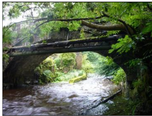
Fig 26: The bridge alongside Bridge End House
