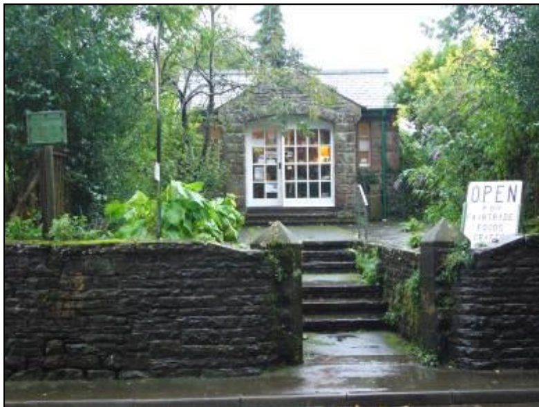
Fig. 12: The Fair Trade shop opposite the Church was built as a memorial to John Peel, to be used as a bus shelter. The open front was later closed in with its present glass door and window when it was converted to use as an Information Centre and Shop
