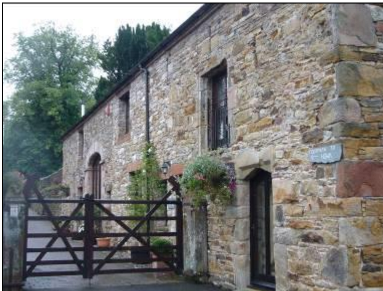
Fig 23 The use of red sandstone to articulate corner, door and window details
