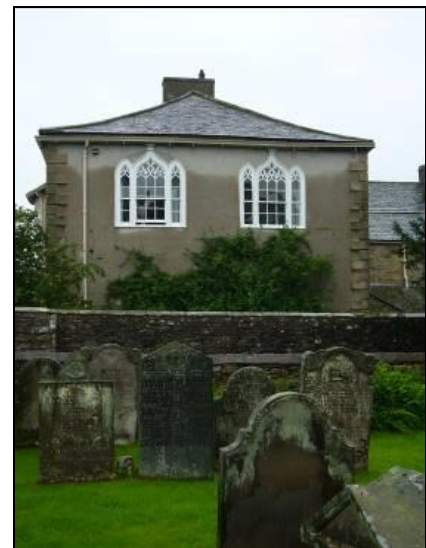
Fig 25: Gothic windows in The Rectory
