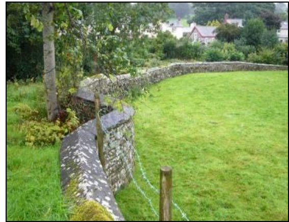
Fig. 17: Riverside walls that following the natural contours of the landscape and curving to avoid large trees
