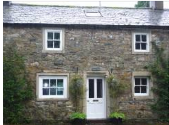
Large, modern rooflights on prominent roofslopes can detract from the character of a historic building. Smaller “conservation style” rooflights are preferable
