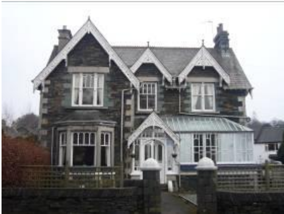
Fig. 35c Finely decorated bargeboards on the front porch and main elevation. Canted bay window with multi-paned upper sashes.
