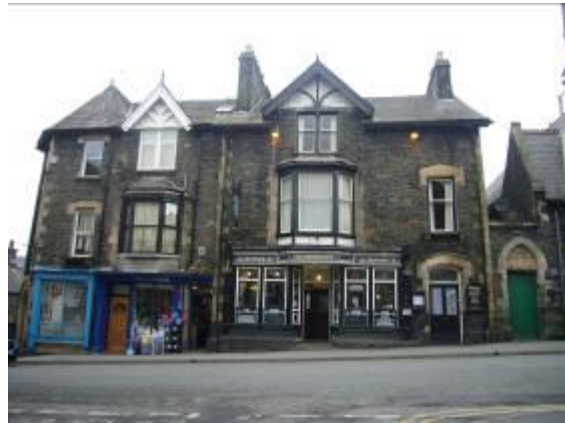
Fig.26 A three-storey Victorian development of shops with two floors of living accommodation above.
