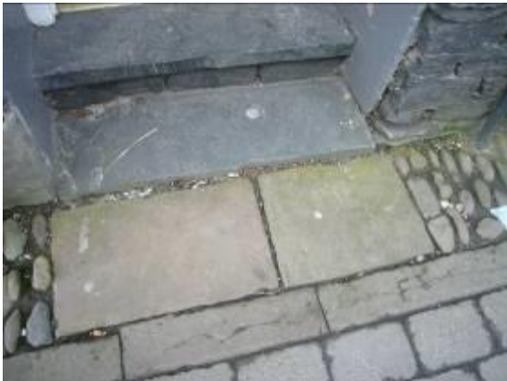
Fig.33 A rare example of historic floorscape in Ash Street.
