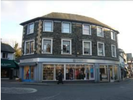
Fig.19 This building has been designed to neatly fit its wedge-shaped site at the end of Ash Street.
