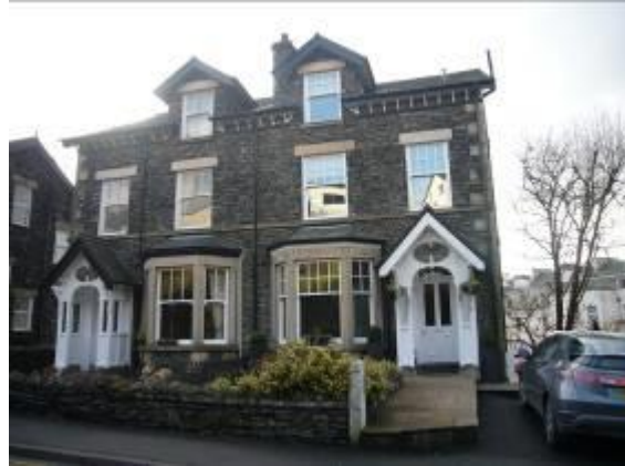
Fig. 35f Ornate matching timber porches, canted bay windows and half-dormers with deep eaves.
