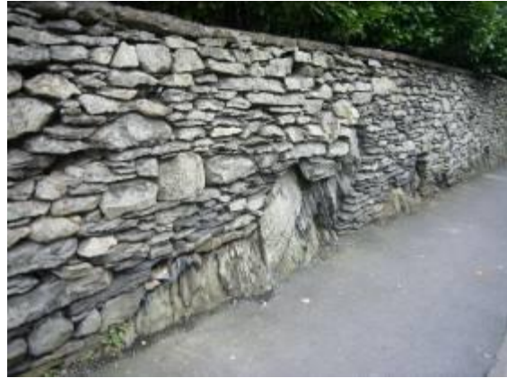
Stone wall built over the bedrock, Biskey Howe Road.
