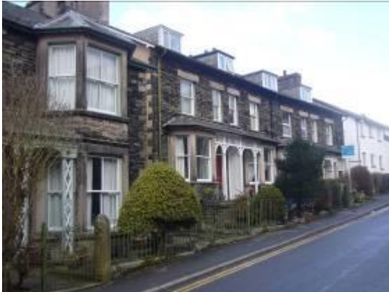
Fig.11 Craig Walk still retains small front gardens and original stone gate-posts.
