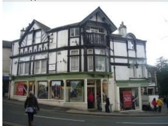
Fig. 35d Deep eaves with exposed rafters. Elegant shopfront. Projecting corner bay with timber balustrade to balcony above.
