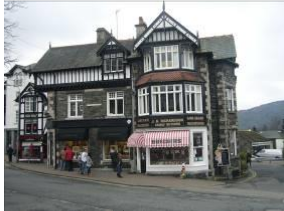
Fig.20 Typical late 19 th century use of local stone (first floor) and applied timbering (second floor).
