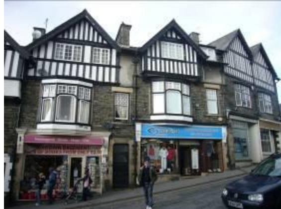
Fig. 35b Carefully detailed first floor overhanging window (oriel). Mix of stone and mock timber-framed upper floor.
