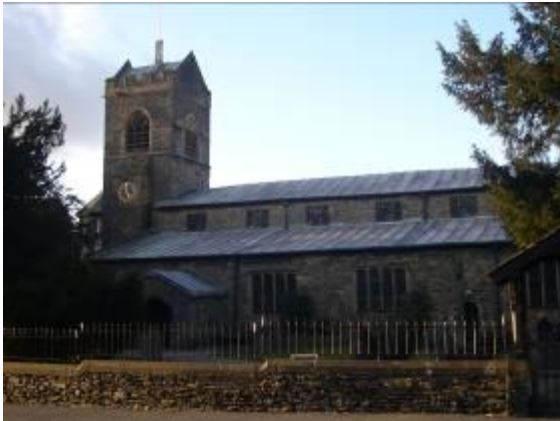
Fig.17 The low-pitched lead-covered roof of St Martin's Church is unusual in the Lake District. Most churches have slate roofs.
