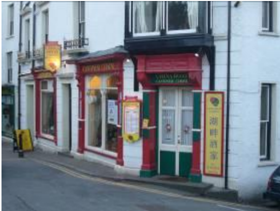
Fig.MP1 Signage needs to be carefully monitored and controlled with regard to size, design and materials to ensure that any negative impact is kept to a minimum.
