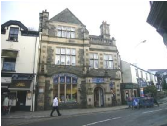
Fig.7 Different types of local stone are combined to great effect on this Victorian building.
