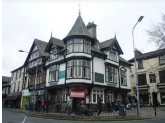
Fig.18 Steep gables and corner turret make this building a landmark feature of the conservation area.
