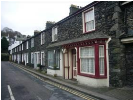
Fig.25 This plain two-storey terrace contrasts markedly with the richly adorned Victorian guest houses nearby.
