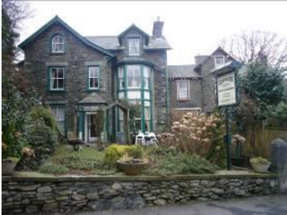
Fig. 35e Local greystone walls with large quoins. Two-storey bay window and steeply pitched half-dormer.
