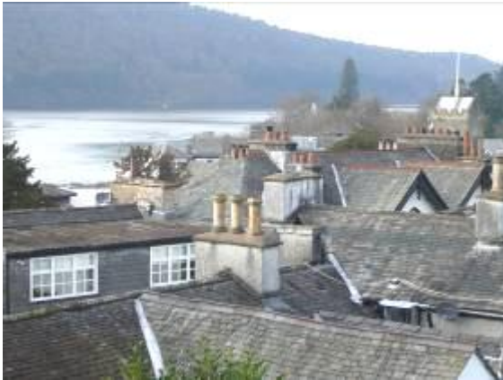
Fig.5 Bowness has a lively roofscape of chimney stacks, pots, ridge tiles and gables.
