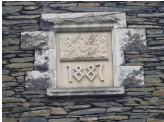
Fig.12b The date is carved into a sandstone block set in a wall of local greystone.
