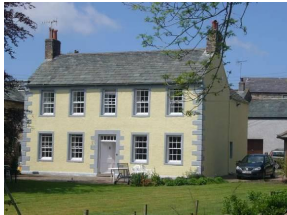
Fig. 32 Blindcrake Hall. This façade has been added to an earlier building. A datestone to the rear reads: 'D & T G 1728'.
