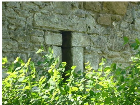
Fig. 8 Narrow slit windows for ventilation are characteristic features of the village's barns.
