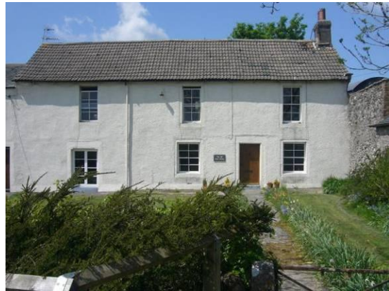
Fig. MP2 Twentieth-century profiled roof tiles have altered the appearance of this 18 th century building.
