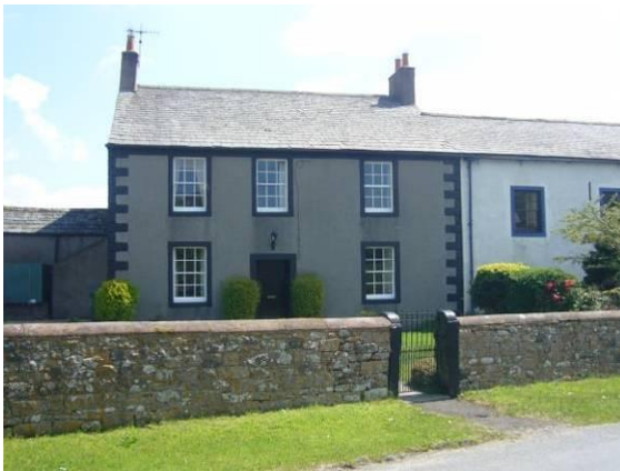
Fig. 31 Croft House, a grade II listed building. Typically, quoins and window surrounds have been highlighted with colour.
