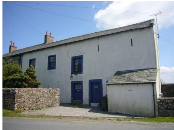
Fig. 38 Windows have been added to this former agricultural barn as part of a residential conversion.
