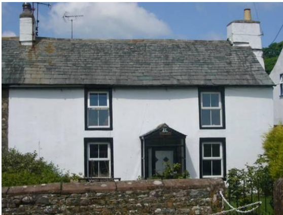
Fig. MP5 This 18 th century building has replacement windows that are obviously modern.
