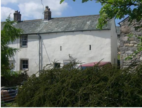
Fig. 33 Ventilation slits in the agricultural part of a longhouse, i.e. a barn and dwelling under one roof.
