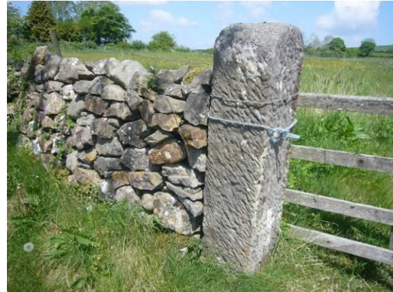
Fig. 2 Limestone walls and gate piers are a typical form of boundary treatment.
