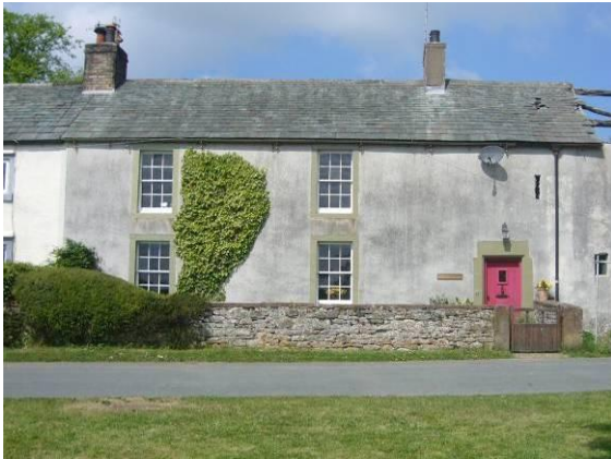
Fig. 18 Low Farmhouse (1729). The front boundary wall is a good example of a limestone wall; the footpath to the front door is cobbled.
