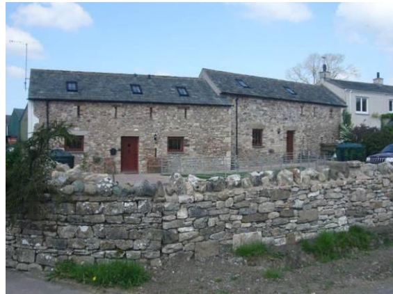
Fig. 15 Former agricultural barns converted to residential use.
