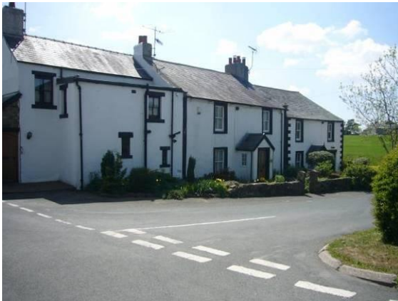
Fig. MP1 The flat-roofed extension to the building on the left, formerly a public house, does not harmonise with the row of cottages.
