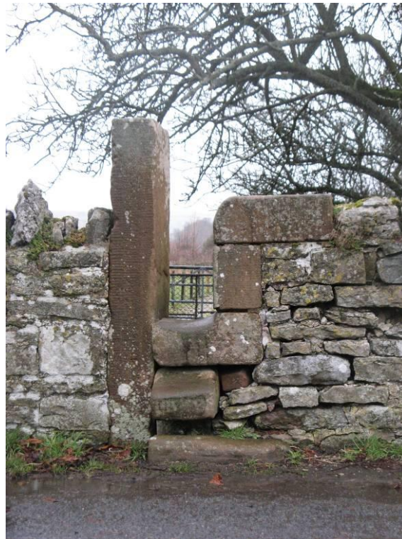
Fig. 12: A distinctive stile constructed from red sandstone. The sandstone would have been imported from the Penrith area.
