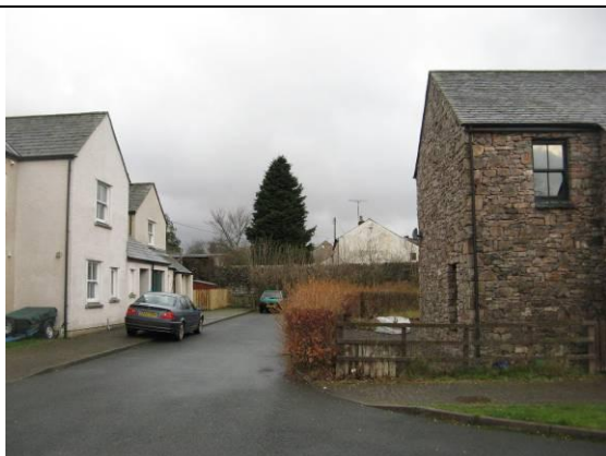
Modern highway treatment at Grange Field.
