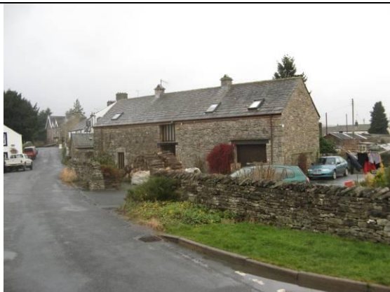
Numerous rooflights inserted into the principal roofslope of historic farm buildings disrupt the integrity of the traditional expanses of unbroken slates.
