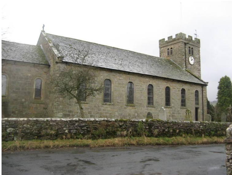
Fig 3: St Patrick's Church (grade II*) is the parish church. It is an important focal building within the village.
