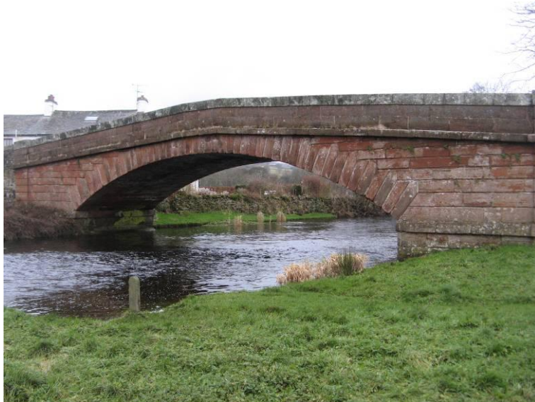
Fig 4: Church Bridge (grade II) is a distinctive red sandstone structure that crosses the River Lowther at the western end of the village.
