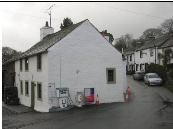
Former house and barn, now the Bridge End Garage.
