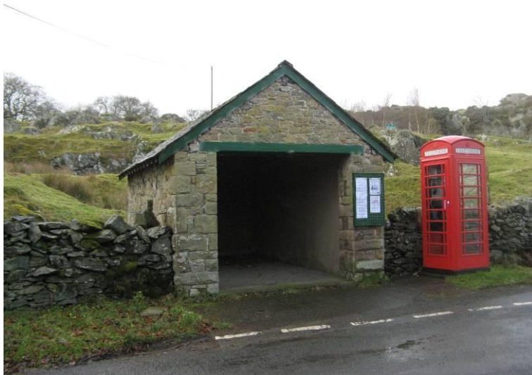
Fig. 10: The red telephone box is an important local landmark on entering the village from the north-west. The rough ground of The Howes rises behind.
