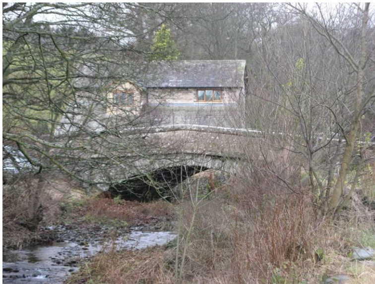
Fig. 1: Bampton Bridge over Howes Beck lies at the centre of the village and is an important landmark in views into the settlement. The Mill, the historic corn mill/saw mill lies on the south bank of the beck.
