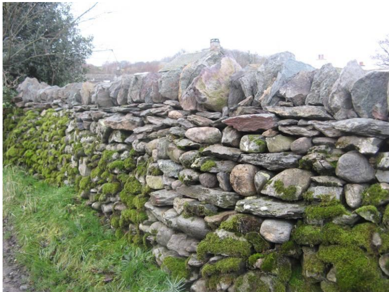
Fig. 9: Rubble stone boundary walls are a distinctive feature of the conservation area.
