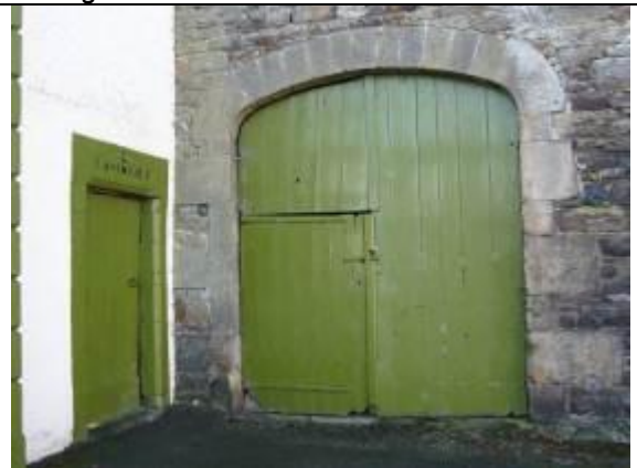
Askham Gate: cart entrance with access door.
