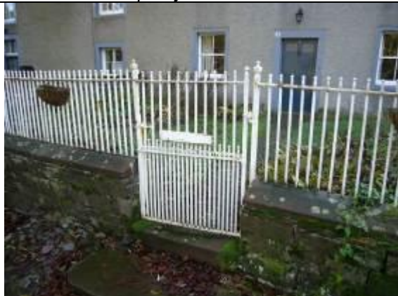
Iron railings and gate to front of Hall Cottage
