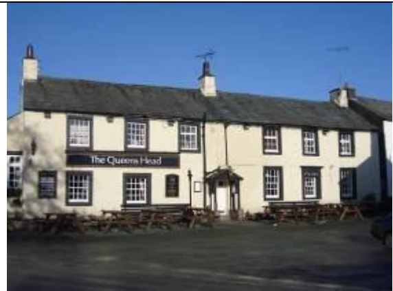
Fig. 12 The Queens Head is an 18 th century building, listed grade II, which may have originated as two separate dwellings.
