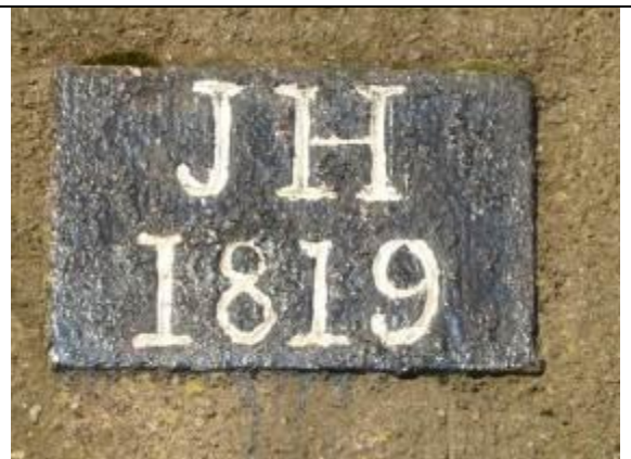
Fig. MP8 Small items and architectural details should be preserved.
