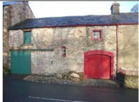
Fig. 20 A typical attached barn, previously used as a butchers, with segmental arched cart entrance and loft door. Note the cobbled surface on the roadside.
