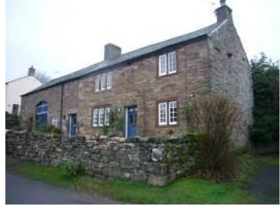
Fig. 10 Unlike the cottage opposite, the stonework of this old farmhouse is currently neither rendered nor limewashed. Historically, it would probably have been limewashed.
