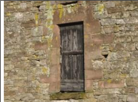
Keld Head Barn: sandstone quins around a loft door.
