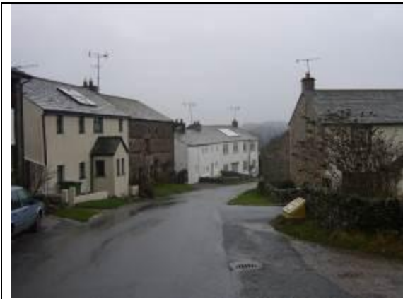
Fig. MP5 Solar panels require sensitive siting on south facing elevations.
