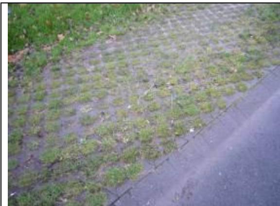
Fig. MP7 Treatment of roadside parking surface needs careful consideration.
