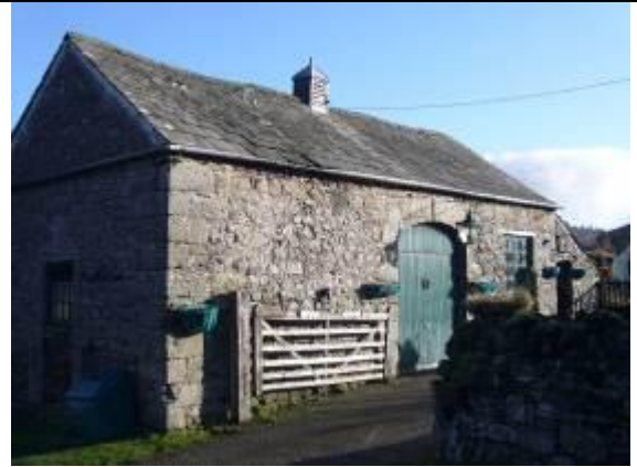
Fig. 40 The former smithy east of Sawmill Cottage has an attractive square vented cupola and is listed grade II.
