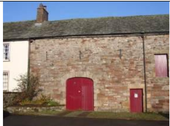
Fig. 38 Cart entrance and vertical slit ventilation holes typical of the area's barns.
