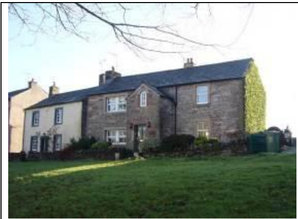
Fig. 15 An old photograph shows that this building was once whitewashed or rendered.
