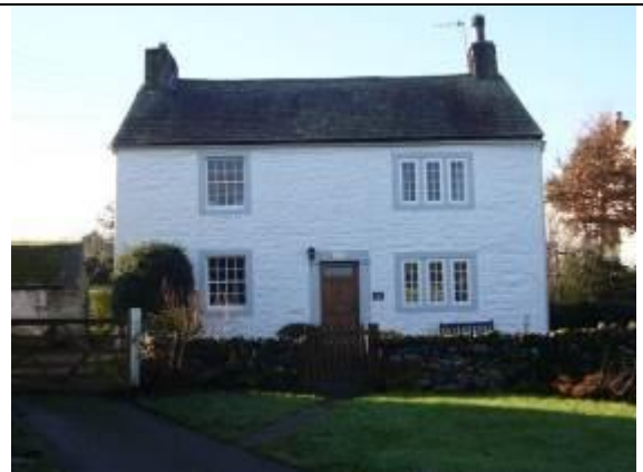
Fig. 6 The Hollies (grade II) has both side-opening mullioned windows and vertical sliding sashes. The house is dated 1800.
