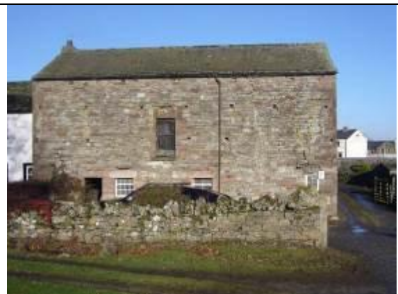
Fig. 34 Stone barn at Keld Head Farm.
