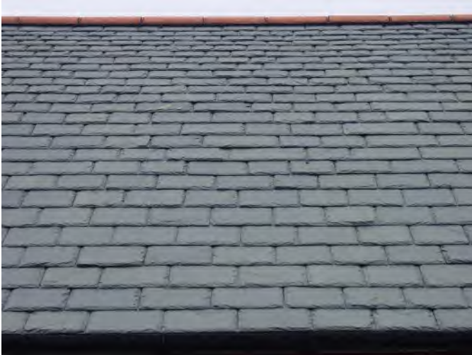
Local blue grey slate is traditionally laid in courses that increase in size towards the eaves. Image: Burlington Slate Ltd
