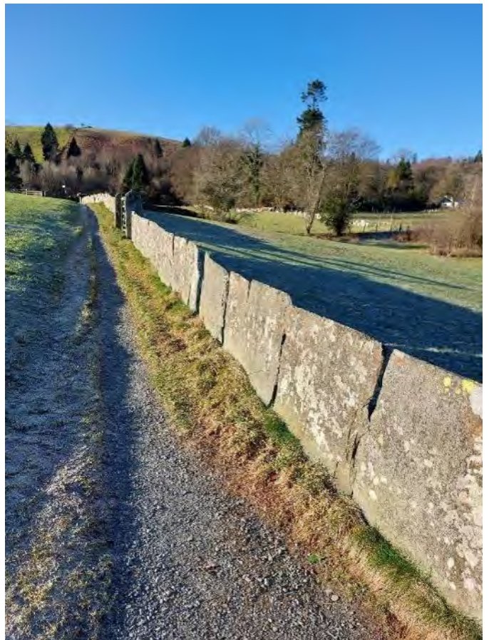
In some parts of the Lake District there are distinctive local boundary traditions, such as this stone slab boundary at Hawkshead.
