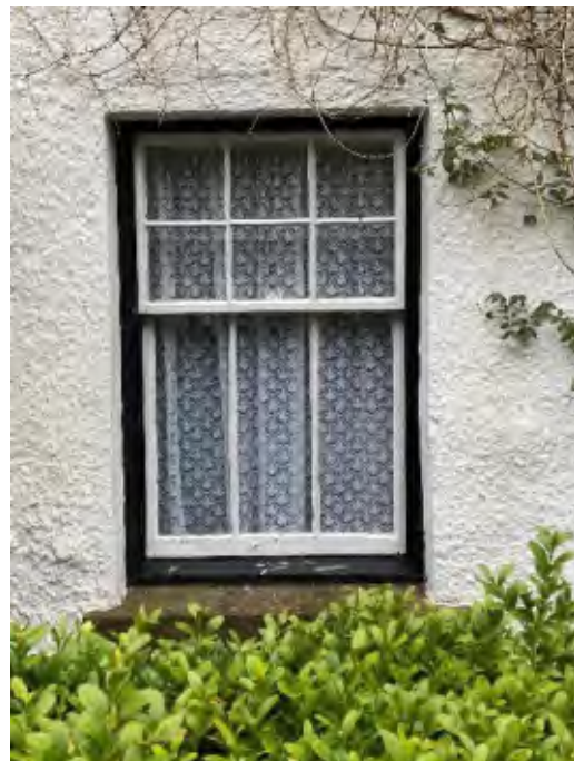
Good quality timber can provide both long-lasting frames and delicate details like these thin glazing bars.
