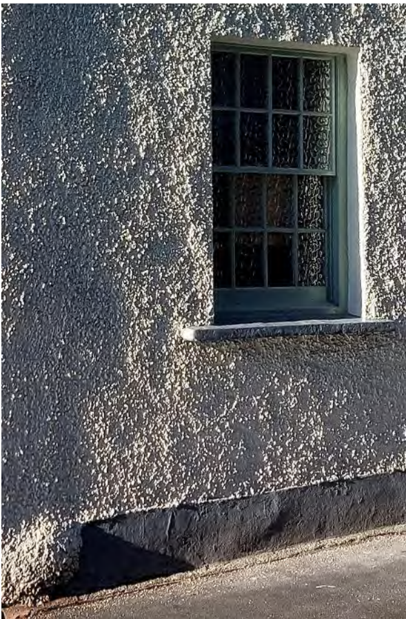
It is called 'roughcast' because pebbles are mixed in with the lime to give a larger surface area for water to evaporate from in wet conditions.
