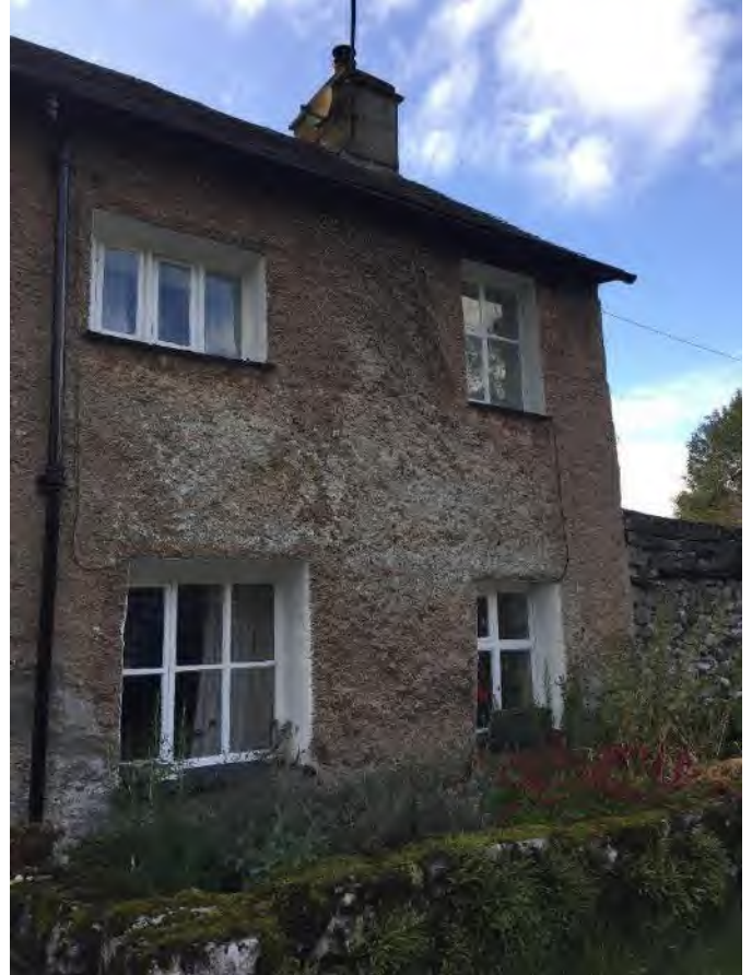
Roughcast render is usually covered by a number of coats of limewash. Here is its bare appearance.
