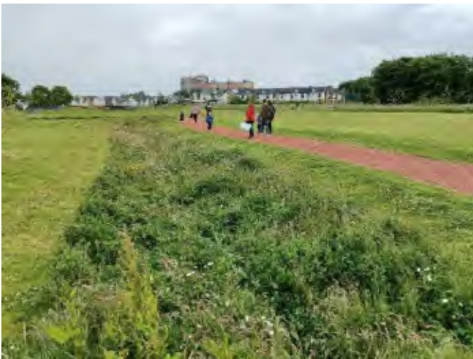
Example of a vegetated swale with soft sides and native species. These types of naturalistic SuDS can be appropriate in rural or settlement edge locations.
