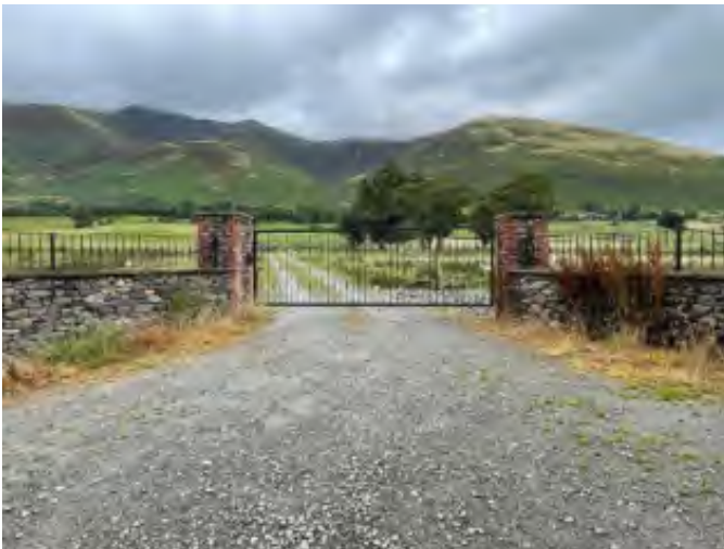
A large, formal-style gateway such as this looks out of place in the landscape due to its suburban character. In this case, the use of imported brick and standard off-the-shelf steelwork exacerbates its visual impact.
