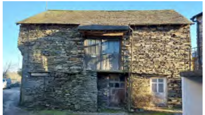
Farm buildings often have a 'rougher' appearance than houses due to the bare stone. Here the external staircase is barely visible against the stonework. Hawkshead
