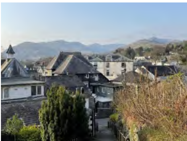
Traditional roofscape in Ambleside requires careful consideration to integrate panels without harming the character.
