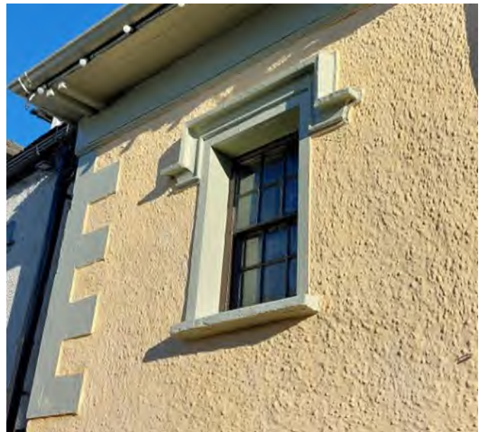
Another lime-based material, roughcast render, was used to cover stone and give a neater looking elevation.
