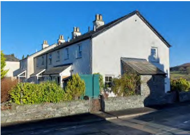
This low wall of Lake District stone is a characterful feature.
