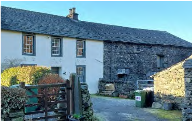
Render finishes were reserved for the higher status buildings, such as this farmhouse, while barns and outbuildings were usually left as bare stone. Borrowdale
