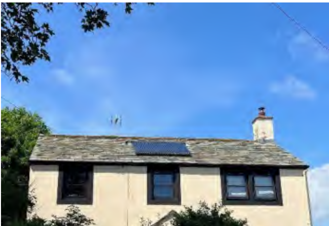
Central placement from the top, bottom, right and left hand edges of the roof makes this thermal water PV panel look less like clutter and means the slate covering still dominates.
