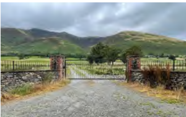
A large, formal-style gateway such as this looks out of place in the landscape due to its suburban character. In this case, the use of imported brick and standard off-the-shelf steelwork exacerbates its visual impact.
