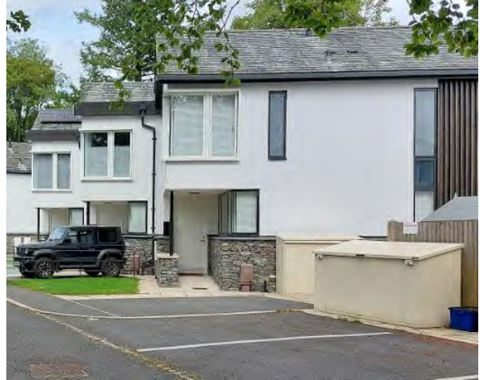
Here the bin stores for a few houses are together in a single collection point.
