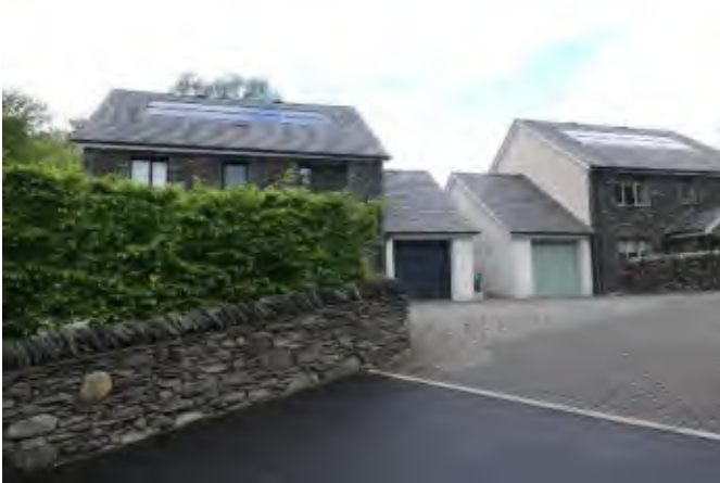
New homes with symmetrically placed in-roof solar panels.
