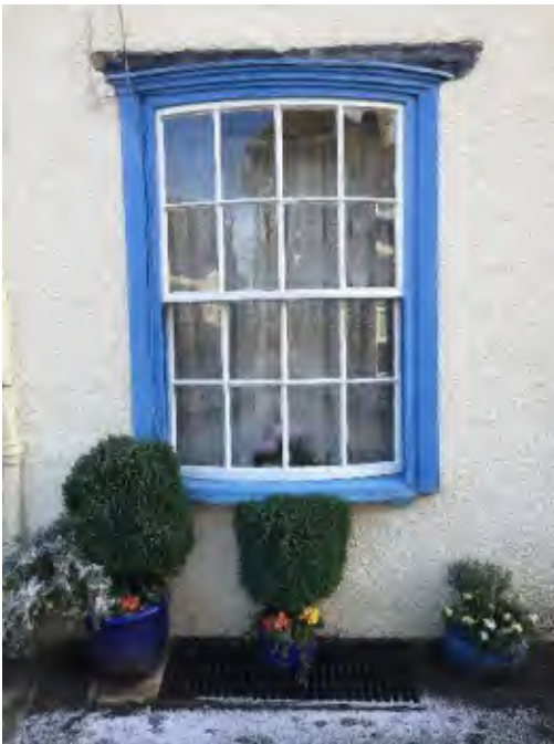
Windows are often referred to as “the eyes” of a building because they make such an impact on its character and appearance.
