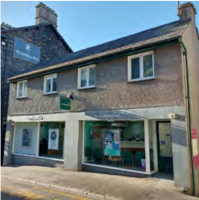
This modern shopfront is minimal in style but has the essential components of a shopfront and makes an important local reference through the use of local stone cladding. The doorway has been sited to provide as level access as possible. Ambleside.
