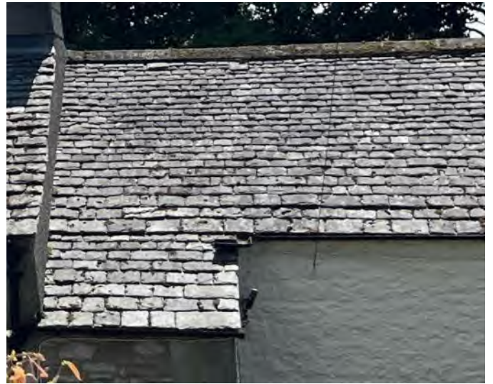
The local green slate is traditionally laid in diminishing courses. In this example the ridge tiles are stone.
