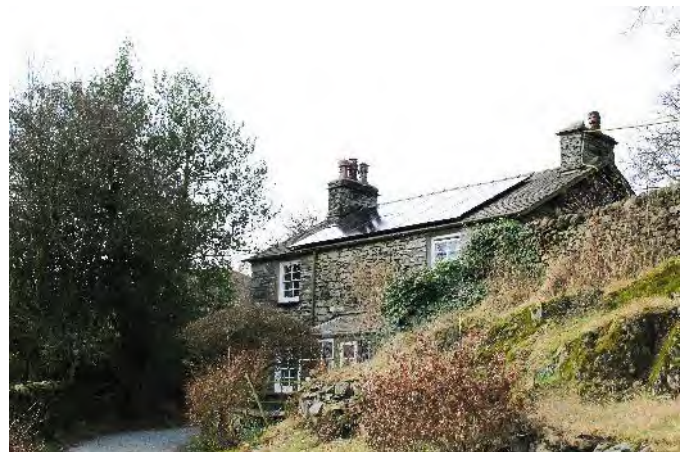
Roof-mounted panels such as these involve the least disturbance to the fabric of the roof and so are preferred for traditional buildings with slate roof coverings.
