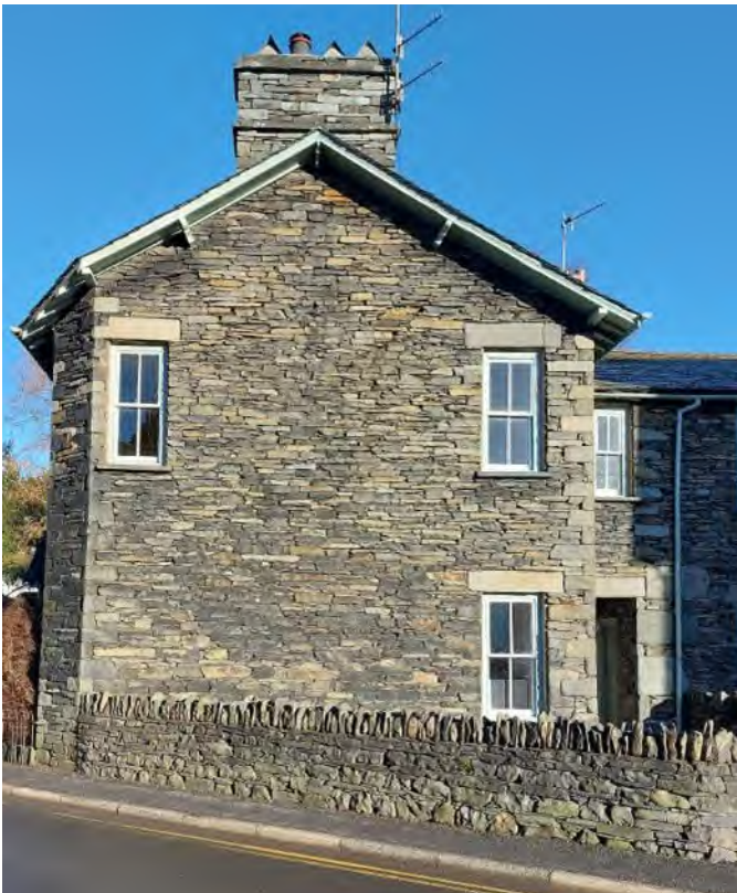
Note the different sizes and shapes of local stone used for the walling of the building, the building corners and the boundary wall.
