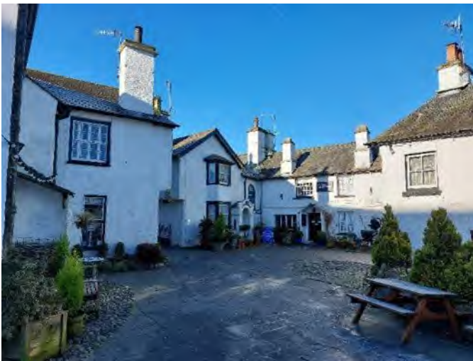
Buildings can join on one or more sides to create enclosed spaces such as this small square. Hawkshead.
