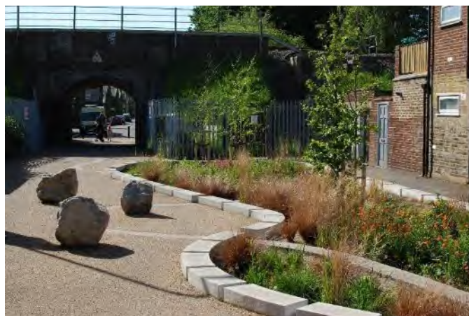
Example of constructed rain gardens with ornamental species which are more suited to town centres.
