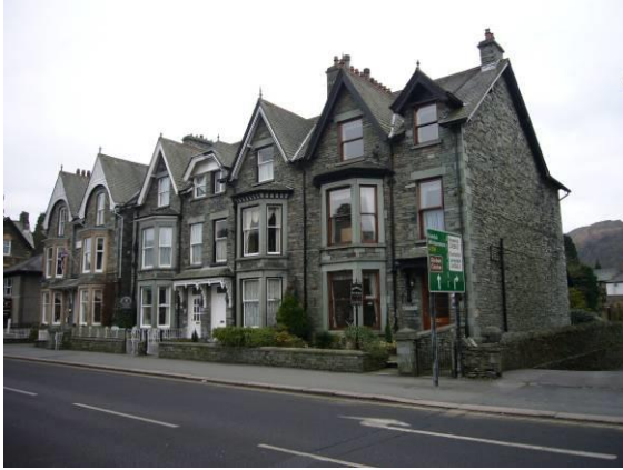
Fig. 20 Gables, ridge tiles, finials, dormers and two storey canted bay windows are typical of the town's Victorian expansion.
