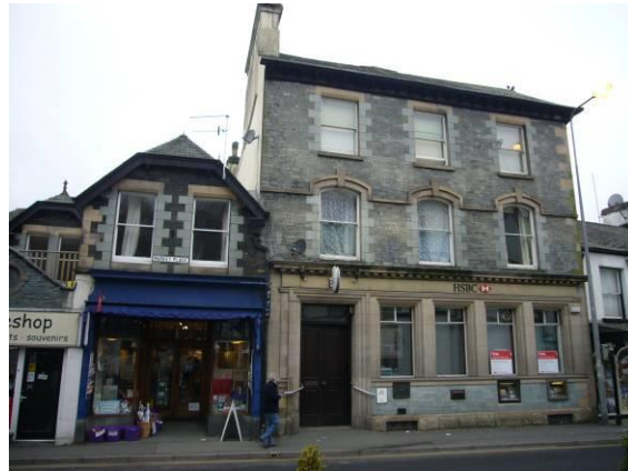
Fig. 33 The ground floor of this Victorian bank building uses an 'imported' brown coloured stone to contrast with the locality's dark greys.
