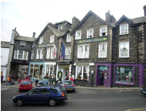
Fig. 3 The Queens Hotel, Market Square displays fine stonework and typically Victorian gables and decorative bargeboards.
