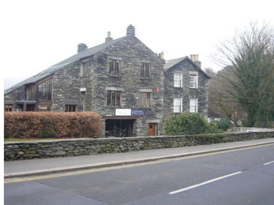
Fig. 17 Former mill building beside Rydal Road.
