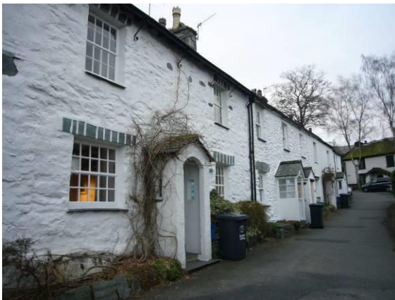
Fig. 12 This row of 18 th century cottages is now listed grade II.
