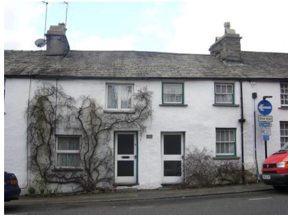
Fig. 41 Altered and enlarged window openings upset the balance of a row.
