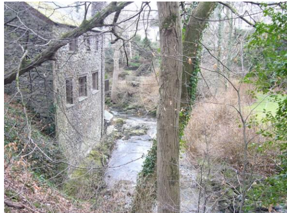
Fig. 8 Stock Ghyll still retains a wild and picturesque character, especially in the eastern part of the conservation area.
