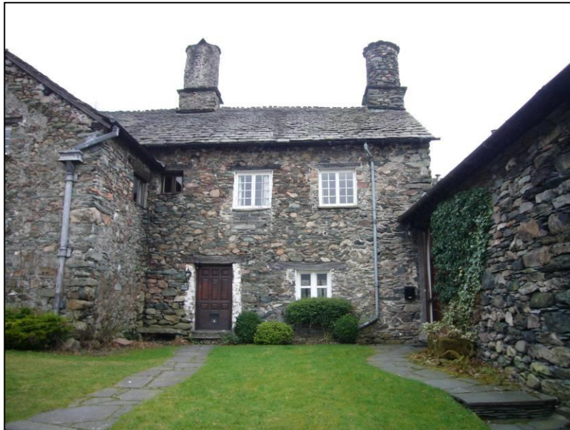
Fig. 9 Howe Head, one of Ambleside's oldest buildings exemplifies Lakeland vernacular by its small square windows, pitched roof, cylindrical chimneystacks and use of local stone for walling and roof.
