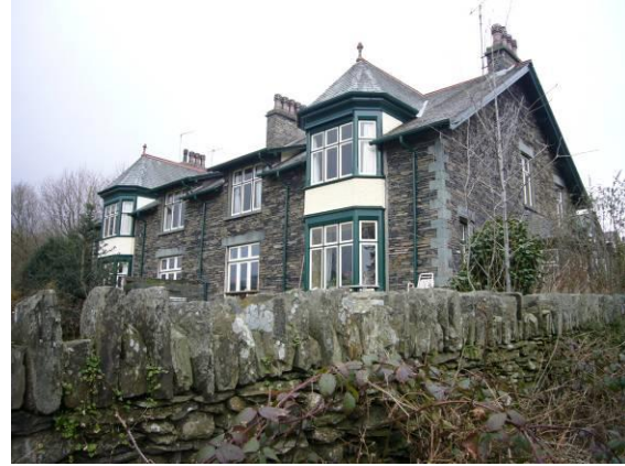
Fig. 21 These semi-detached houses in The Millans turn their back to the road in order to take advantage of the views to Loughrigg Fell.
