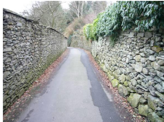
Fig. 29 Nook Lane, an old westward route out of the town, is bounded by high stone walls.
