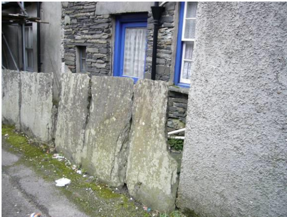
Fig. 28 Stone slab wall to the rear of Corbrig and Planetree House.
