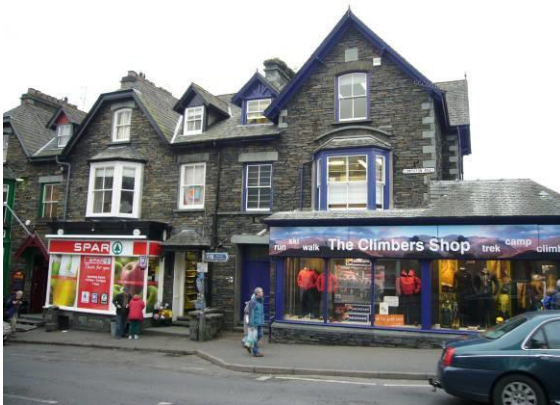
Fig 40 Garishly coloured fascia sign (left) mars the appearance of the host building.
