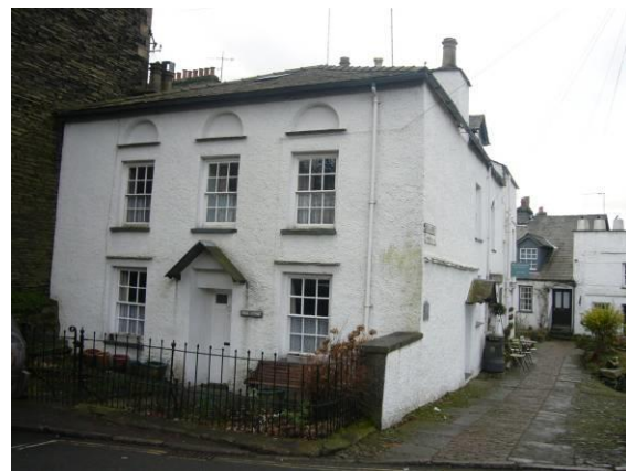
Fig. 4 Stock Cottage, North Road. A Georgian frontage to a colourwashed stone rubble building with slate roof (grade II).
