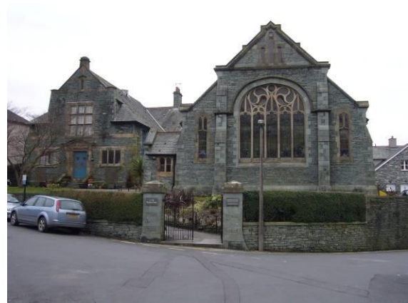
Fig. 36 Former Wesleyan Chapel, The Millans – a building of special character.
