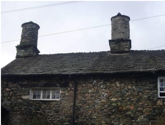
Fig. 32 Howe Head - cylindrical stone chimney stacks and stone flag roofs are particular features of vernacular Lakeland buildings.
