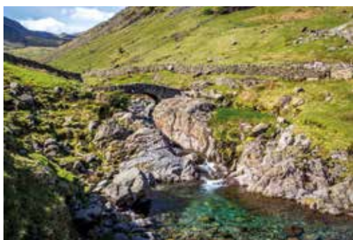
FIGURE 9.10 Stockley Bridge, crossing Grains Gill in upper Seathwaite. A classic example of a small, single-arched Lake District packhorse bridge.
