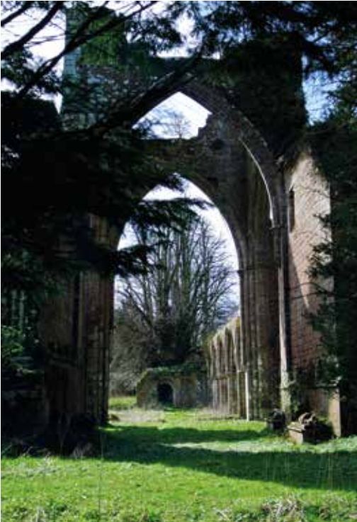
FIGURE 7.8 The remains of the church tower at Calder Abbey
