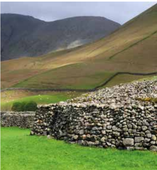
FIGURE 6.8 A clearance wall forming part of the ancient field system at Wasdale Head. Here the walls are widened into clearance cairns to accommodate the huge amount of stone that has been transported from the fellsides by water.
