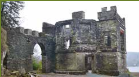
FIGURE 5.9 Claife Viewing Station prior to restoration
