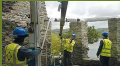
FIGURE 5.10 The restoration of Claife Viewing Station
