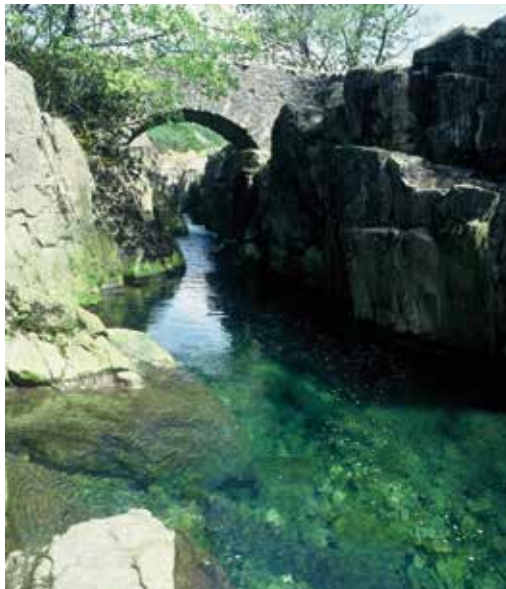
FIGURE 4.11 The single span stone packhorse bridge at Birks, crossing the River Duddon
