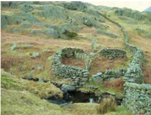
FIGURE 4.13 Sheepfold and sheepwash of drystone and slate shard construction at Stephenson Scale
