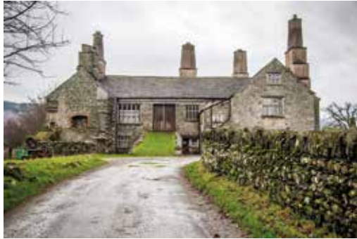
FIGURE 3.11 Coniston Hall, displaying massive, cylindrical chimneys typical of large Lake District houses of the Statesmen period (late 16th/early 17th centuries). The house was later converted to a bank barn and the entrance ramp can be seen in the centre of the building.
