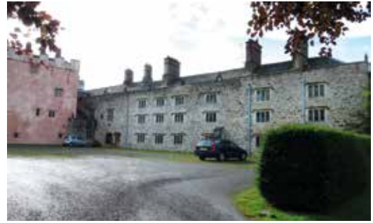
NO. 2 FIGURE 2.c.9.4 Isel Hall
