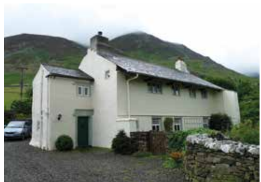
NO. 4 FIGURE 2.c.8.6 Low Hollins Farm
