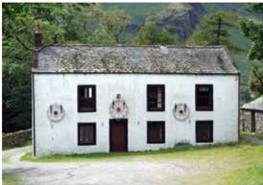
NO. 5 FIGURE 2.c.8.7 Gatesgarth Farm
